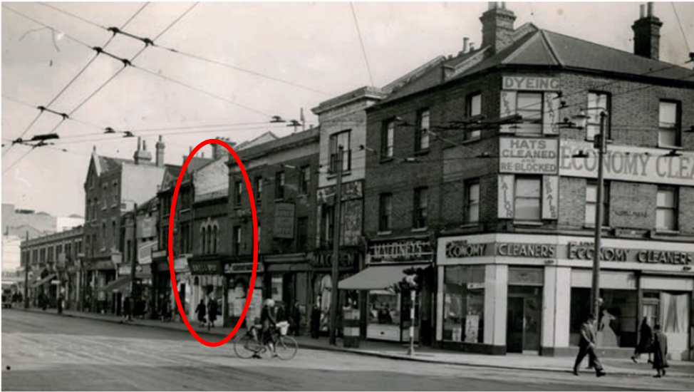
1950s Photograph (No. 410 circled) (Source: Haringey Council)
