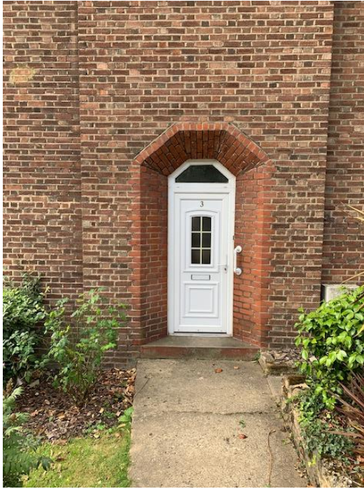
P 2: Existing front door and brick surround around flat 3. The brick surround design will be re-used around the proposed new entrance.
