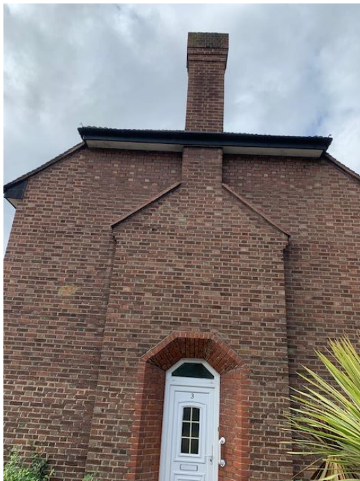
P 3: Existing chimney stack on the front of the building which will be recreated on the front of the new extension.
