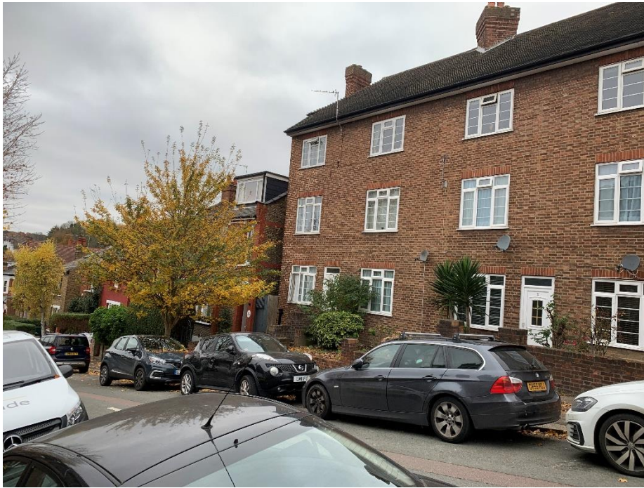
Elevation to Alexandra Gardens looking towards No 39
