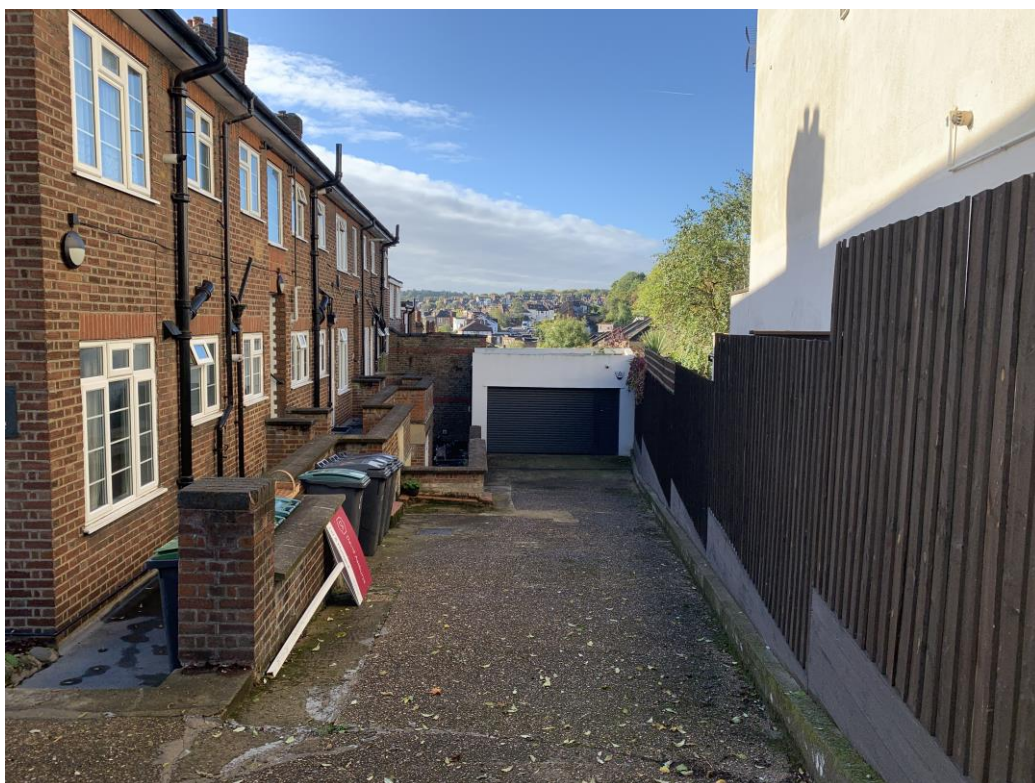
Rear elevation with view towards existing garage
