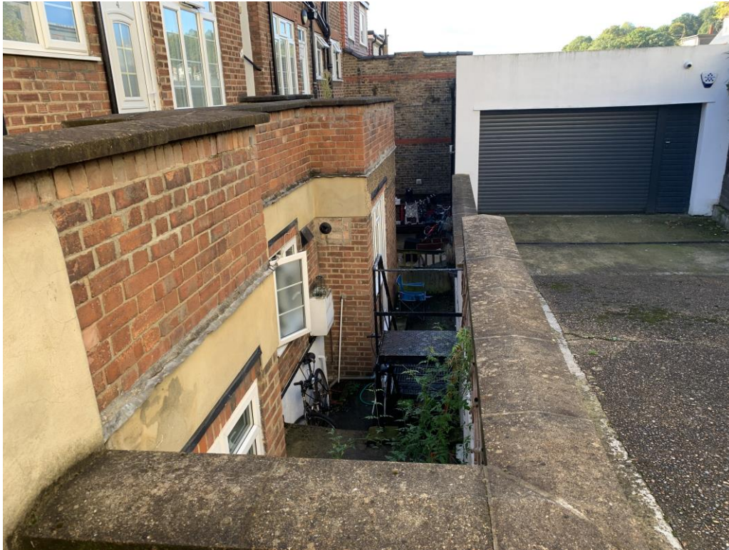
Existing lightwell to rear with external staircase
