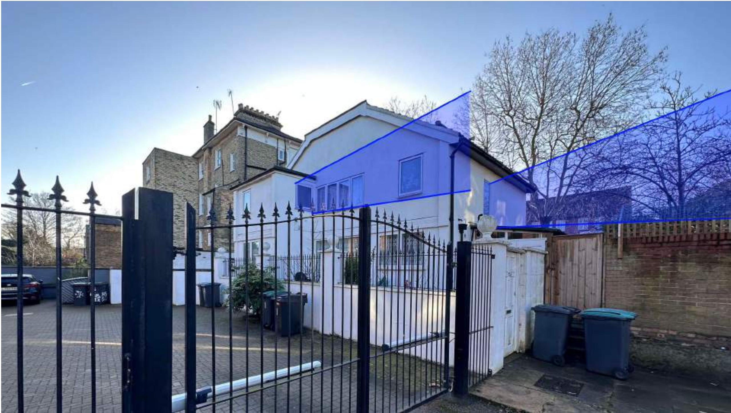
Existing Rear View showing existing windows to rear gardens at 1 - 5 Sussex Gardens.
