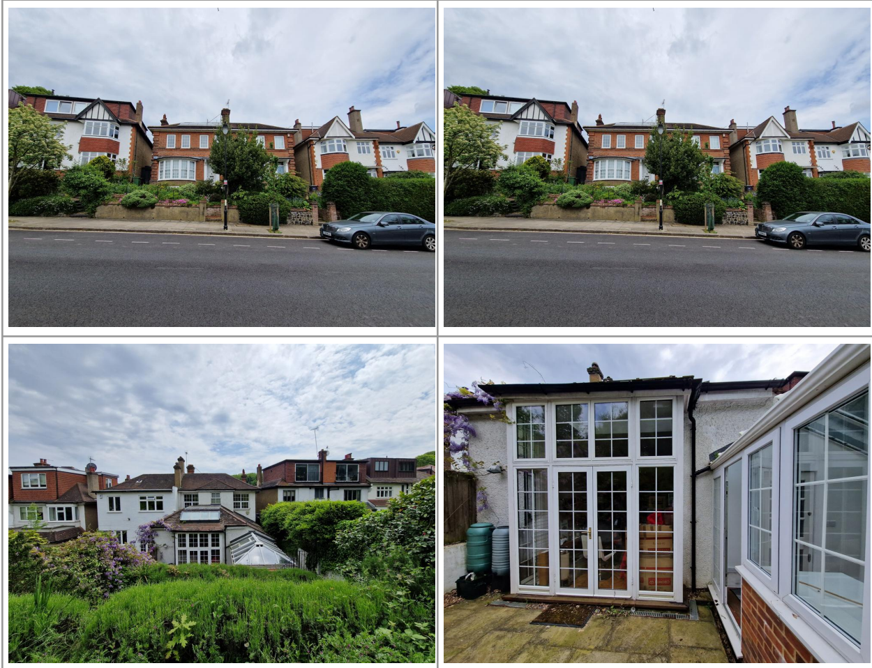
1.1 Above a views of the current house
