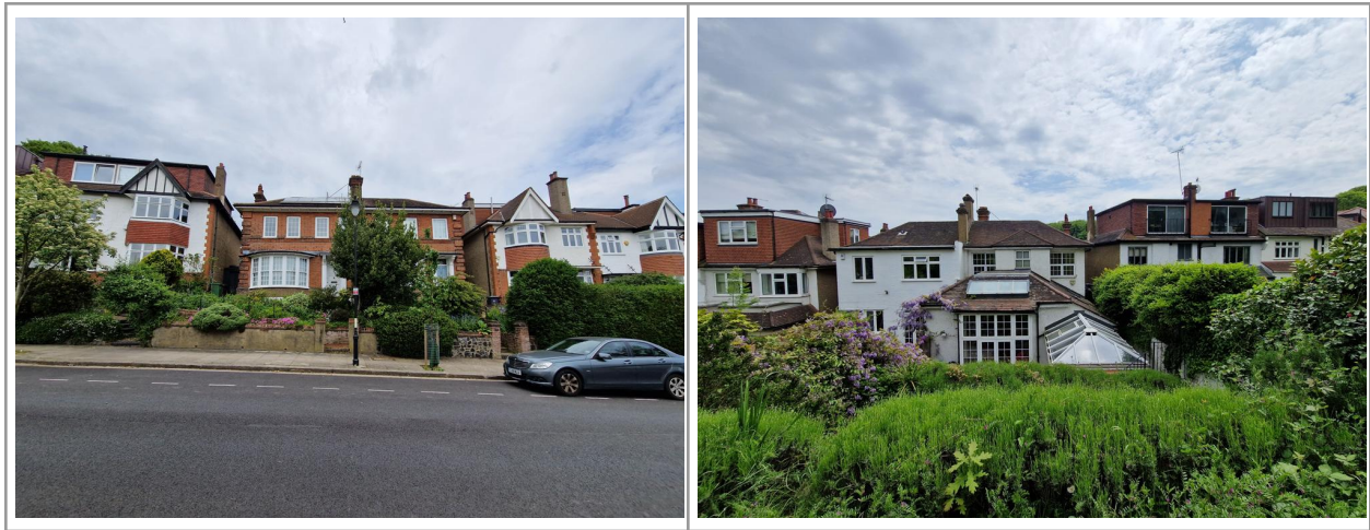
1.2 Above views of the current property
