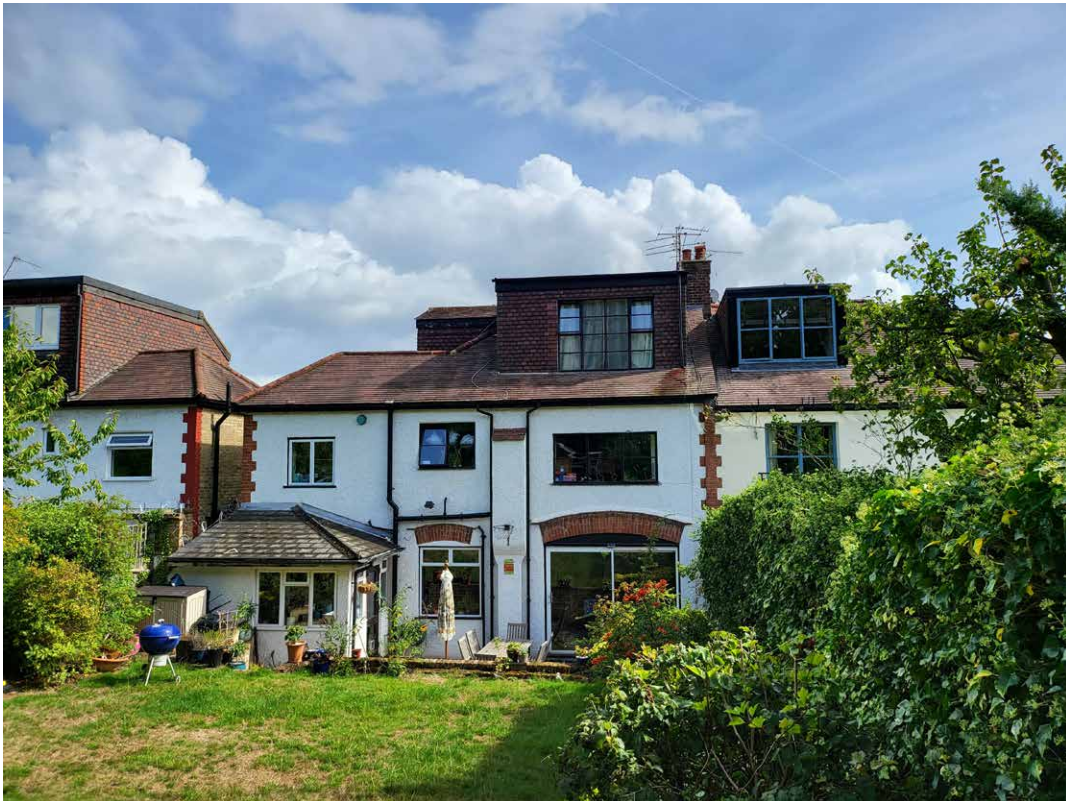
3. Photo showing garden elevation, with existing utility projection seen to the left.
