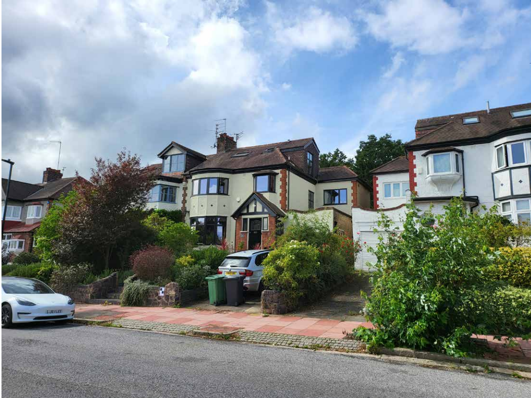
2. Photo showing street elevation.
