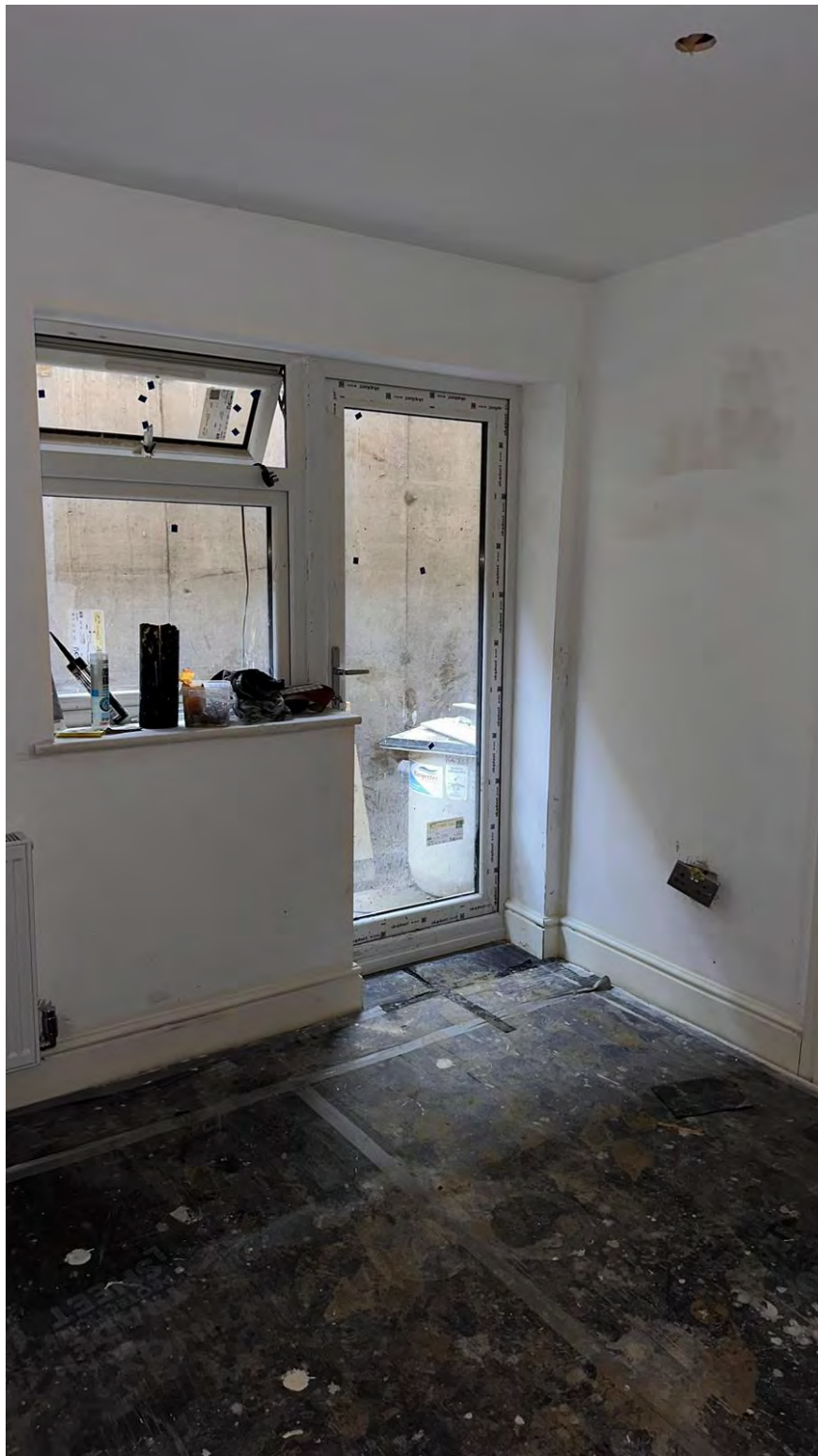
Interior image of lower ground bedroom door/window leading to courtyard/lightwell
