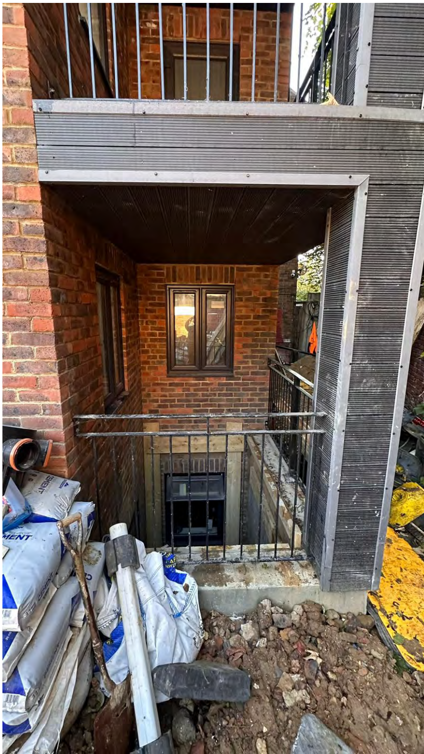
Exterior image at street/ground floor level of rear lightwell (view from north-west)
