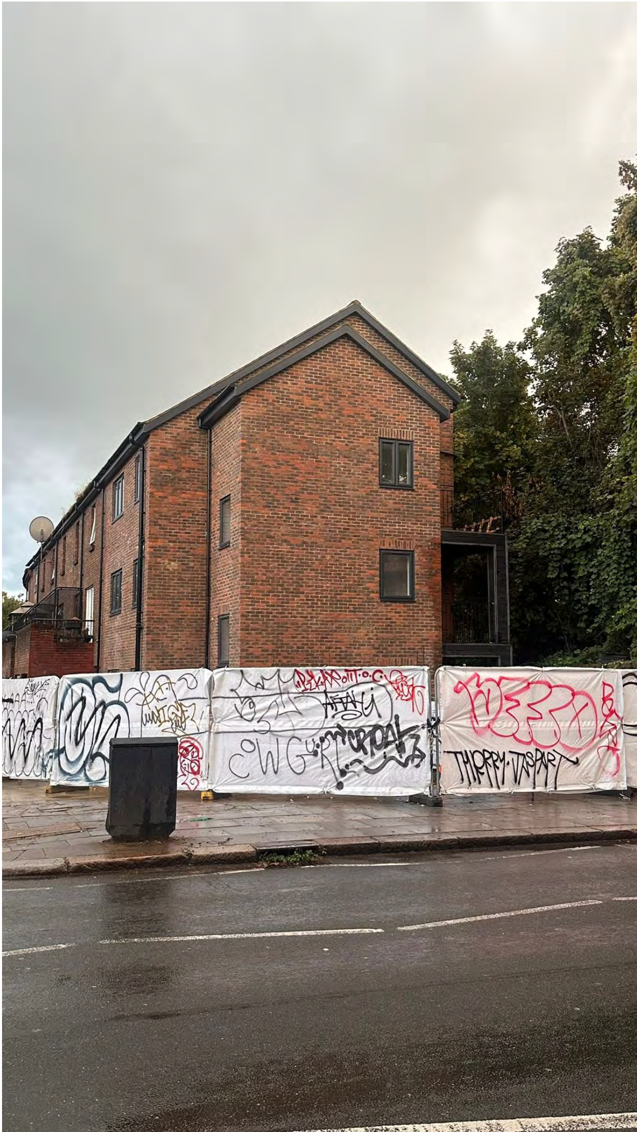
Exterior image of flank elevation, detached end (facing north-west)
