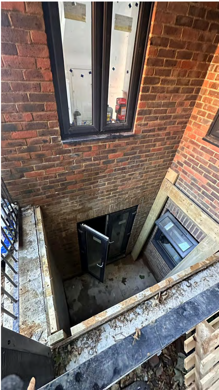
Exterior image at street/ground floor level of rear lightwell (looking down from south-west)
