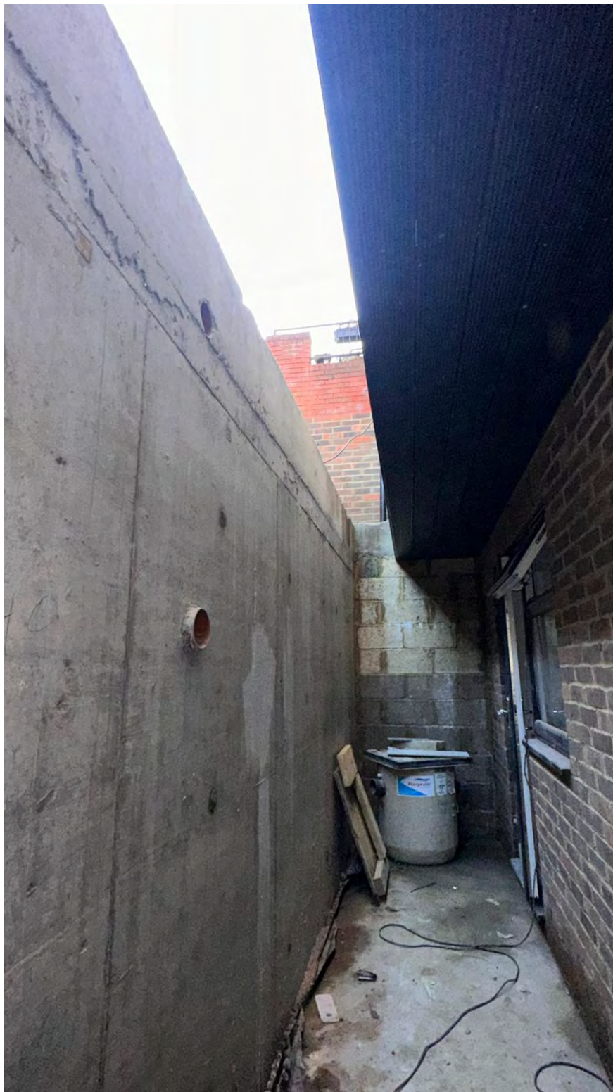
Exterior image at lower ground floor level of front lightwell/courtyard (view from north-west)
