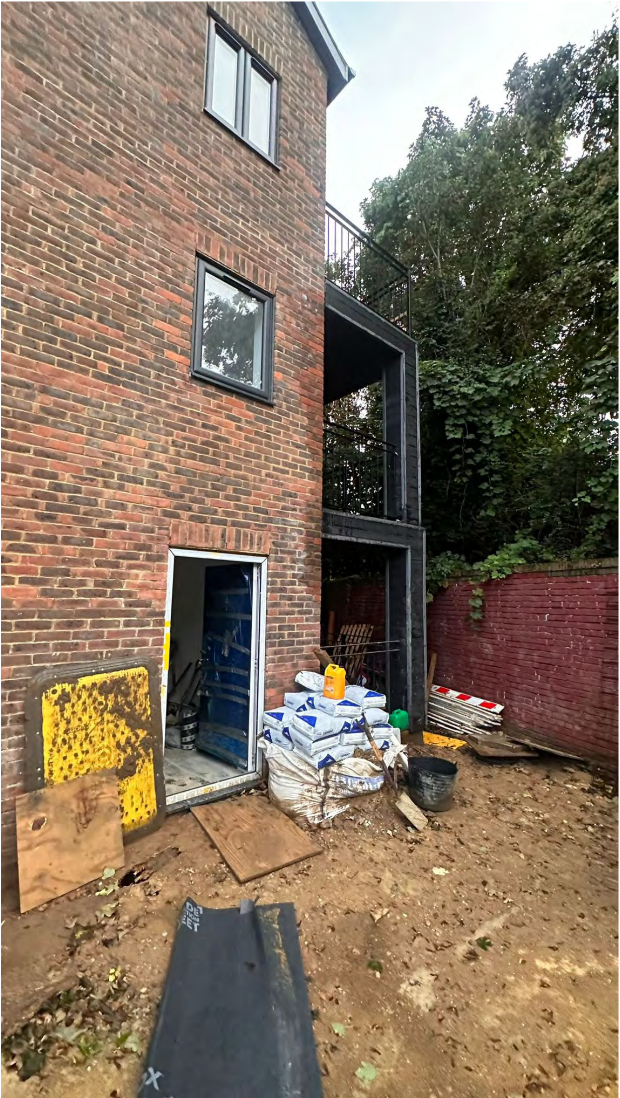
Exterior image of communal entrance to flats, detached end (facing north-west)
