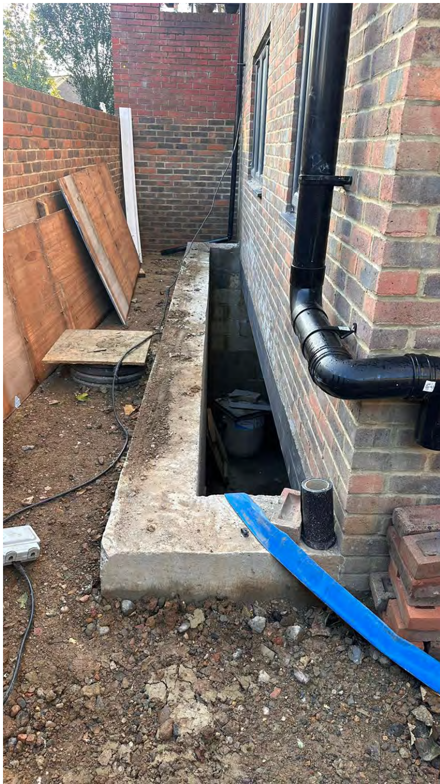
Exterior image at street/ground floor level of front lightwell (view from north-west)
