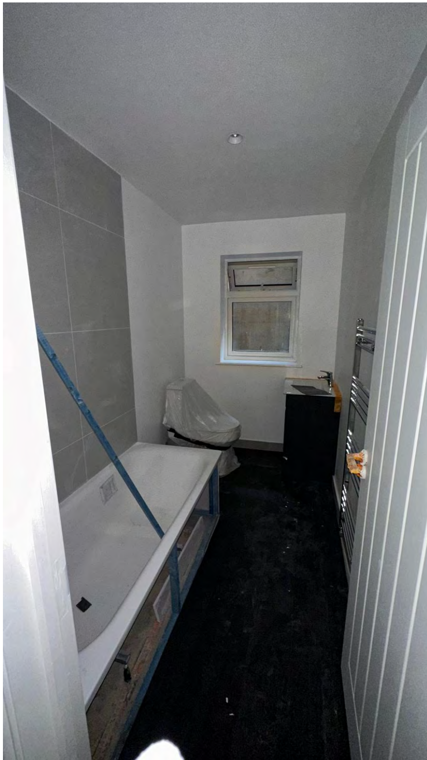
Interior image of lower ground bathroom showing window facing courtyard/lightwell
