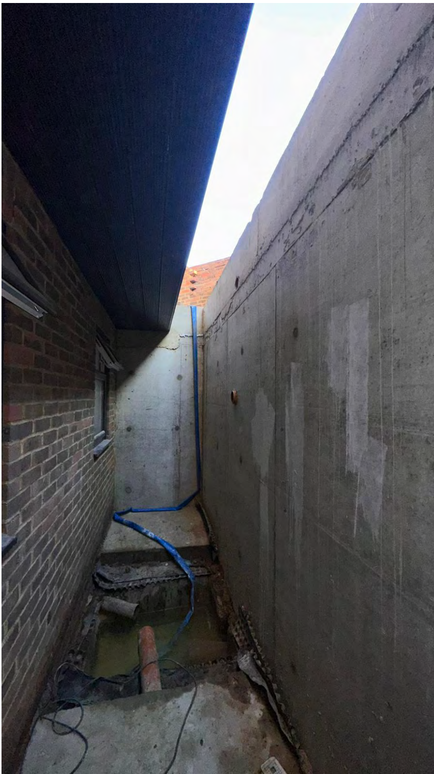
Exterior image at lower ground floor level of front lightwell/courtyard (view from south-east)
