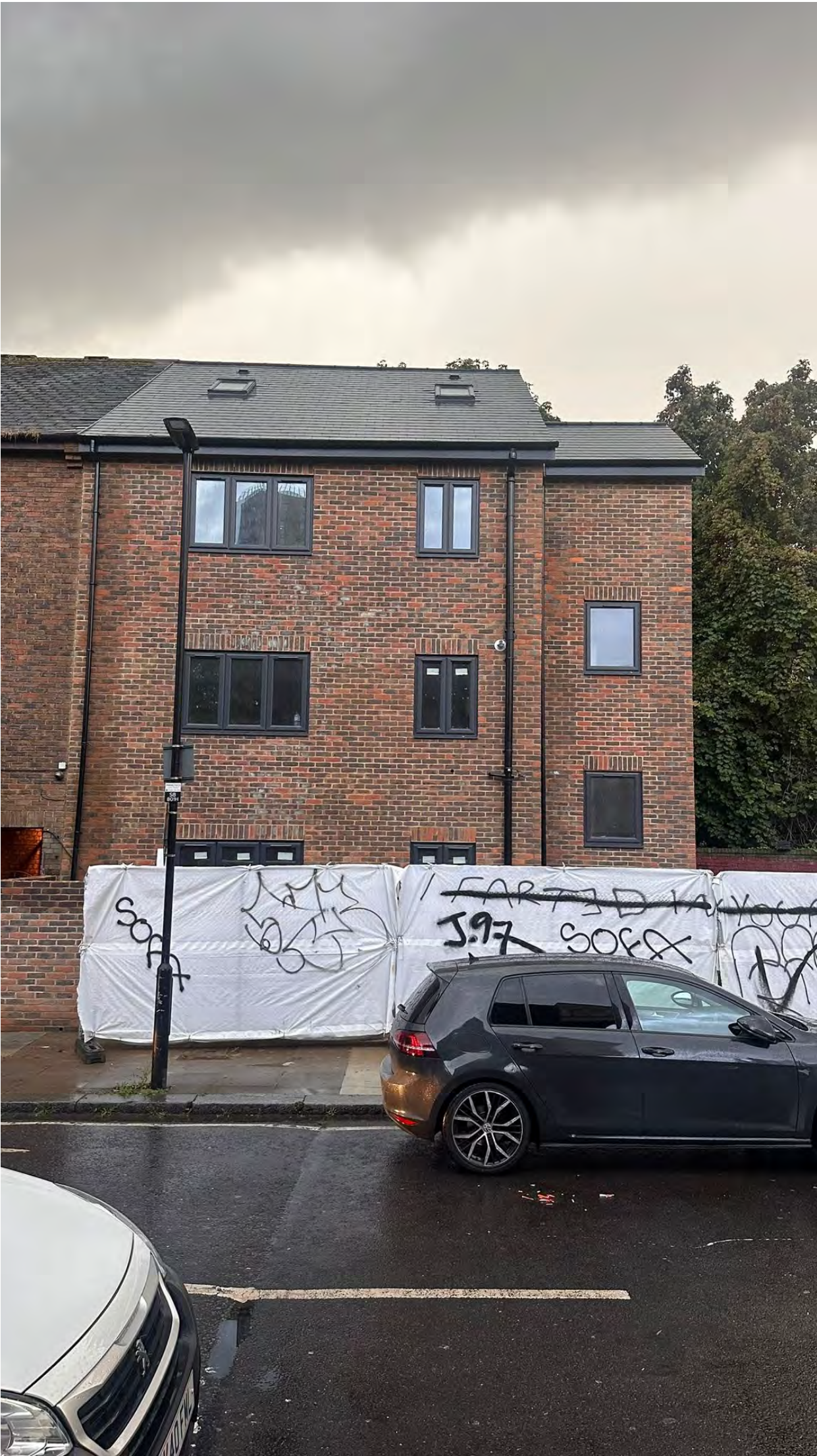
Exterior image of front elevation (facing north-east)
