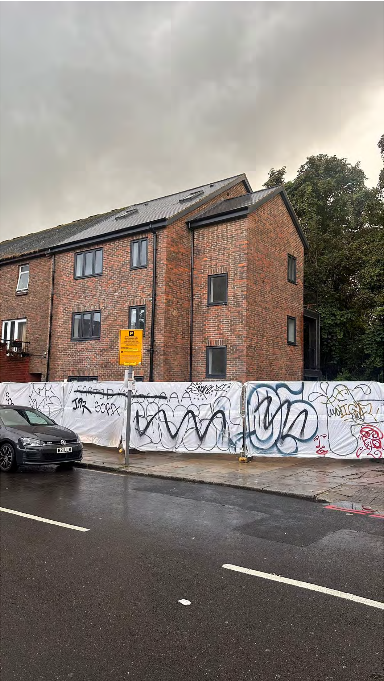
Exterior image of front corner elevation (facing north)
