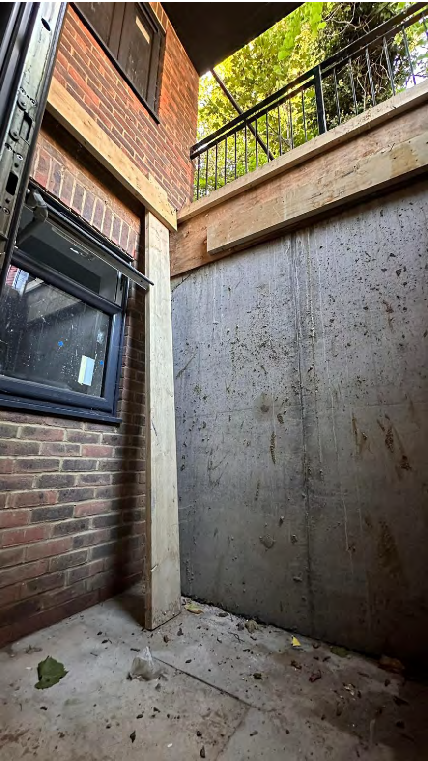
Exterior image at lower ground floor level of rear lightwell/courtyard showing bathroom window (view from east)
