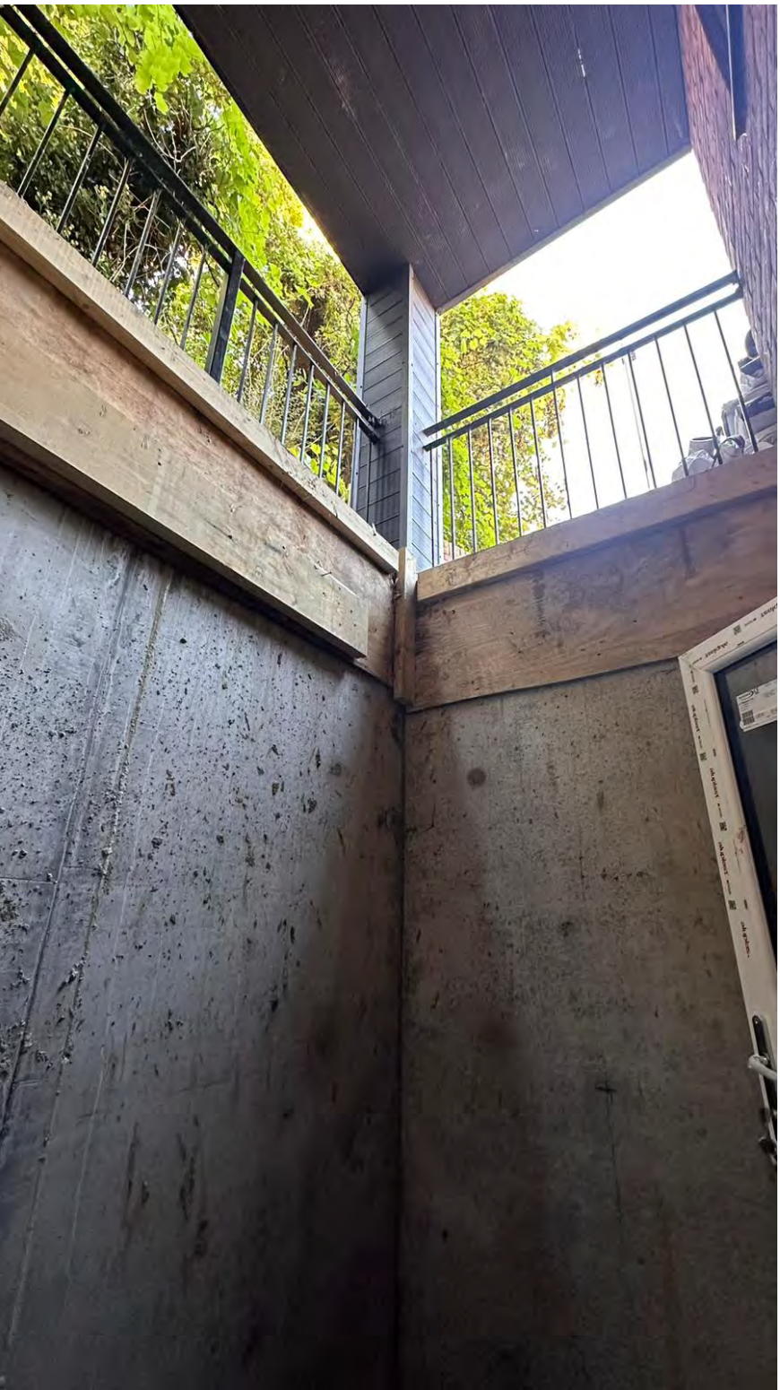
Exterior image at lower ground floor level of rear lightwell/courtyard (view from west)
