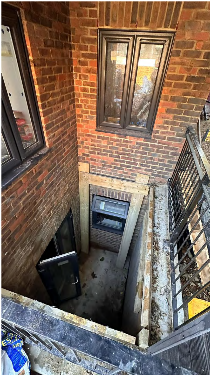
Exterior image at street/ground floor level of rear lightwell (looking down from north-west)
