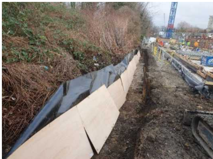
Image 33: Root Barrier Works
