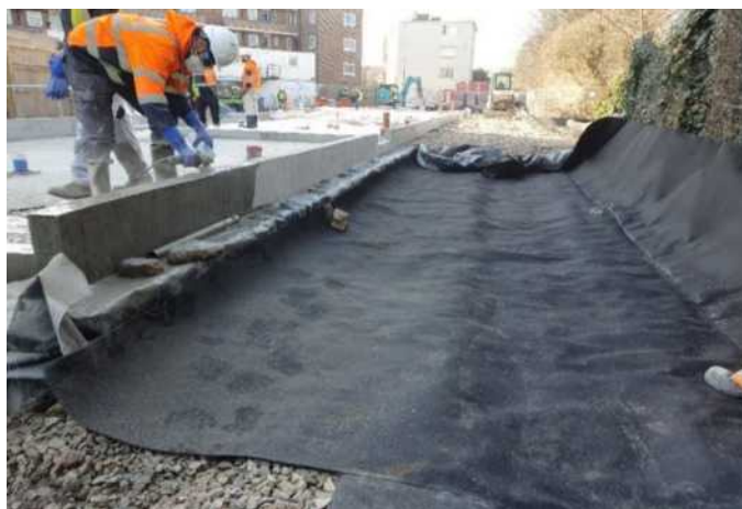
Image 40: Root Barrier Works
