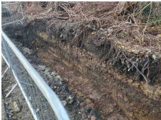
Image 33: Root Barrier Works
