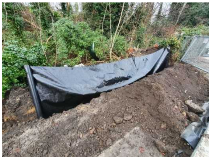
Image 37: Root Barrier Works
