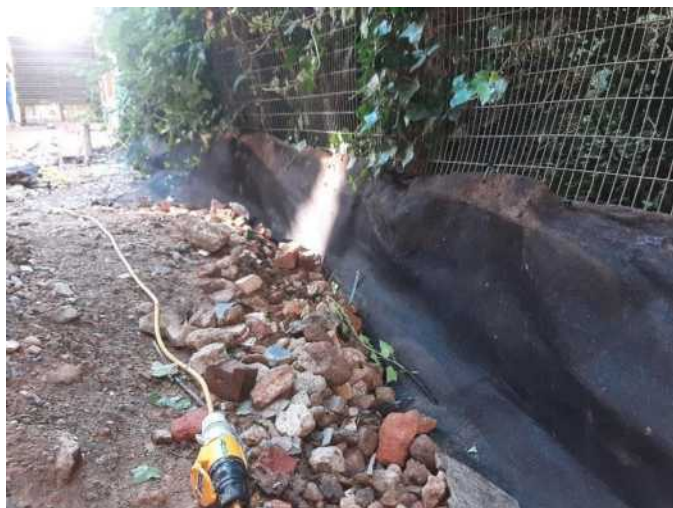
Image 466: Root Barrier Works
