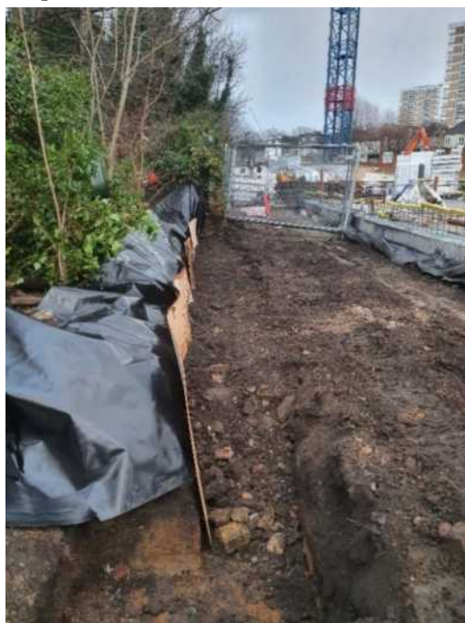
Image 39: Root Barrier Works
