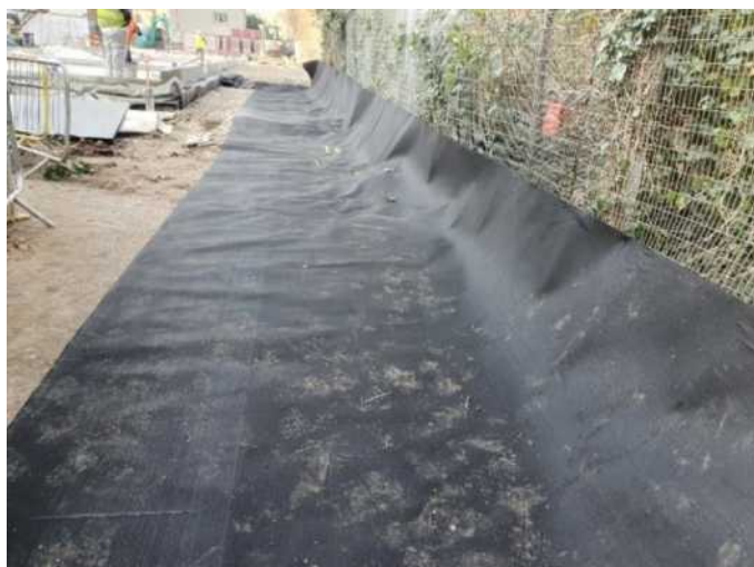
Image 43: Root Barrier Works
