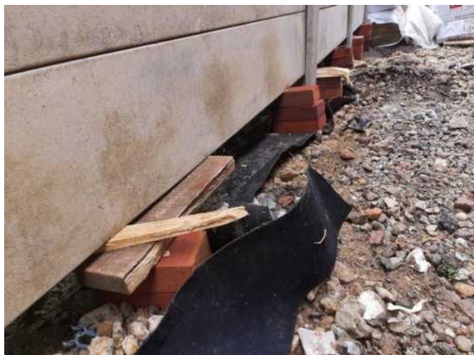
Image 45: Root Barrier Works
