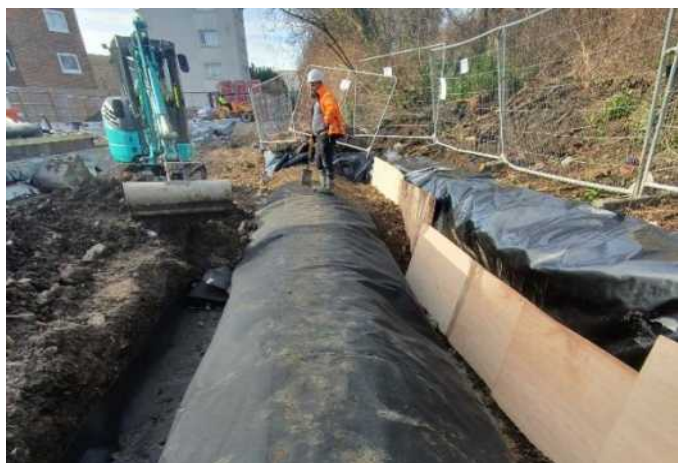
Image 39: Root Barrier Works
