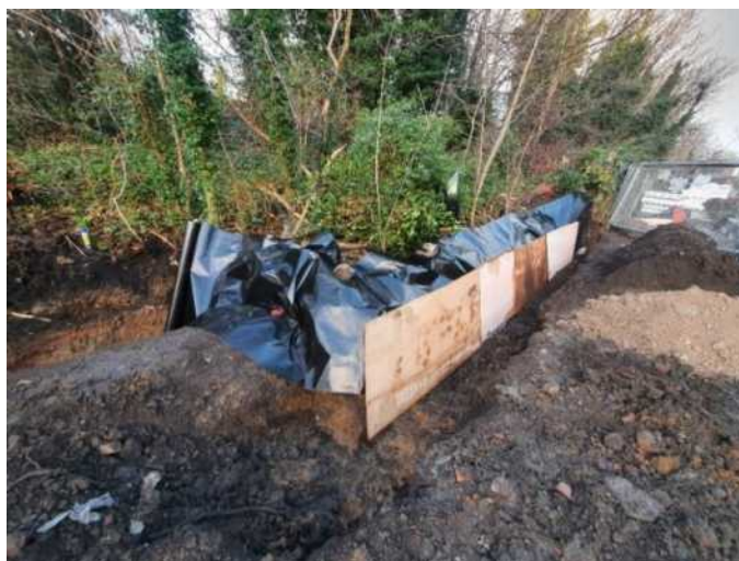
Image 38: Root Barrier Works
