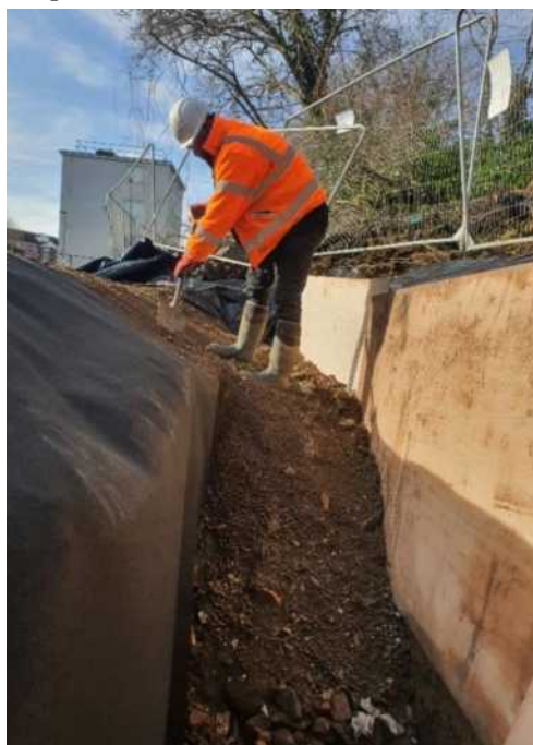
Image 40: Root Barrier Works
