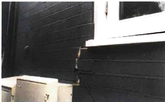
Crack to front left brickwork.
