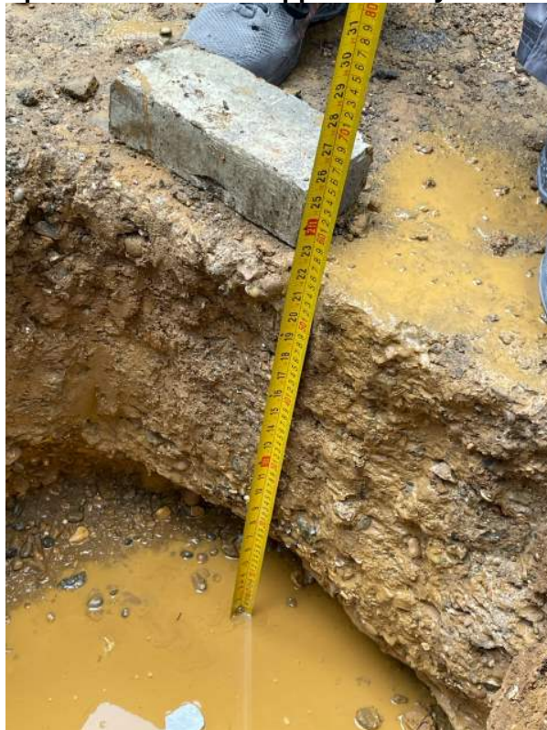
Existing foundation exposed
