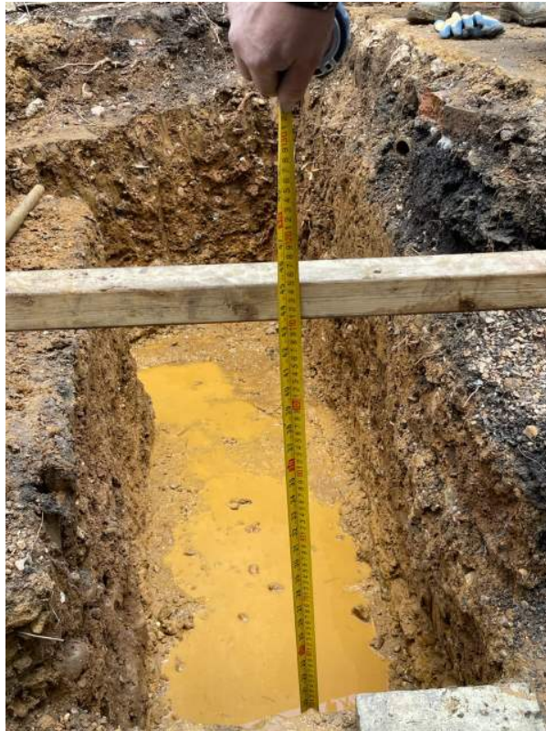
Depth of excavations approximately 1100mm
