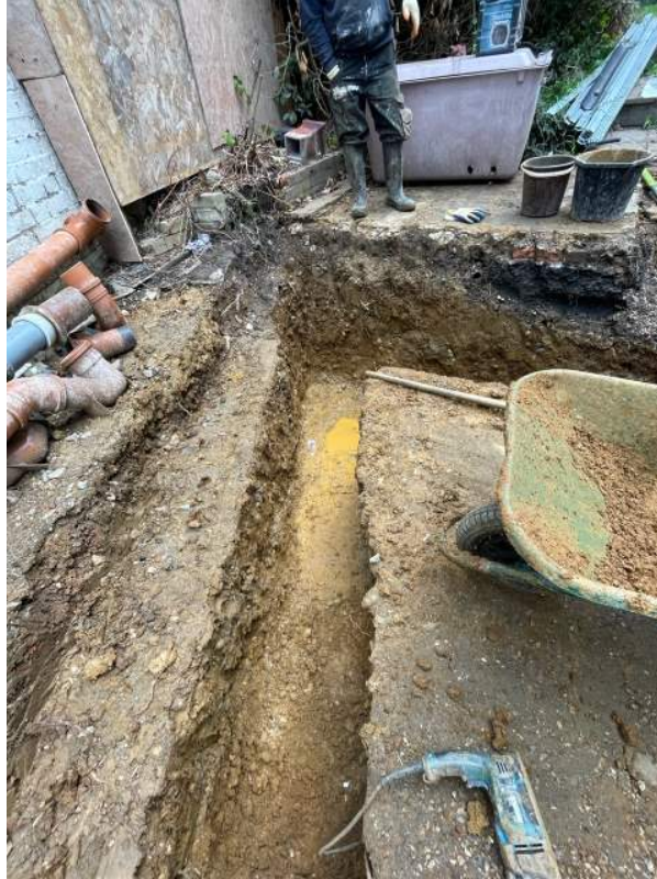
Excavation alongside neighbouring house
