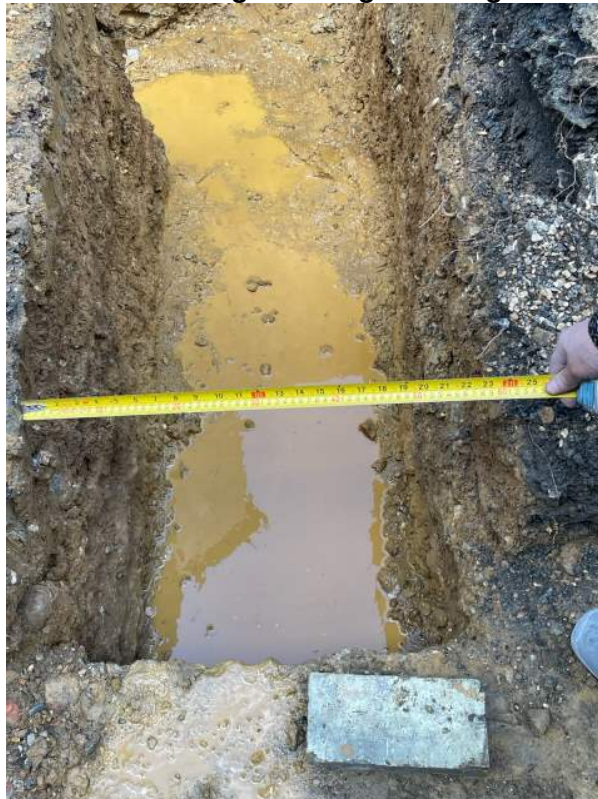
Excavation approx 600mm wide - ground water to the bottom of the excavation
