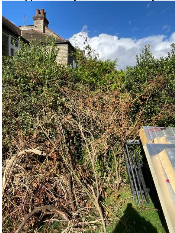
Possible coniferous tree approximately 5-7 metres away from the foundation
