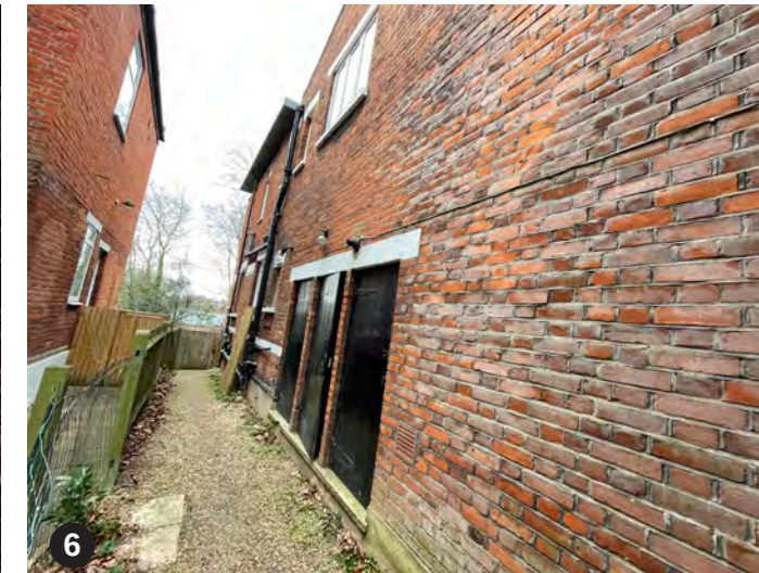
6 East facade path/ route
