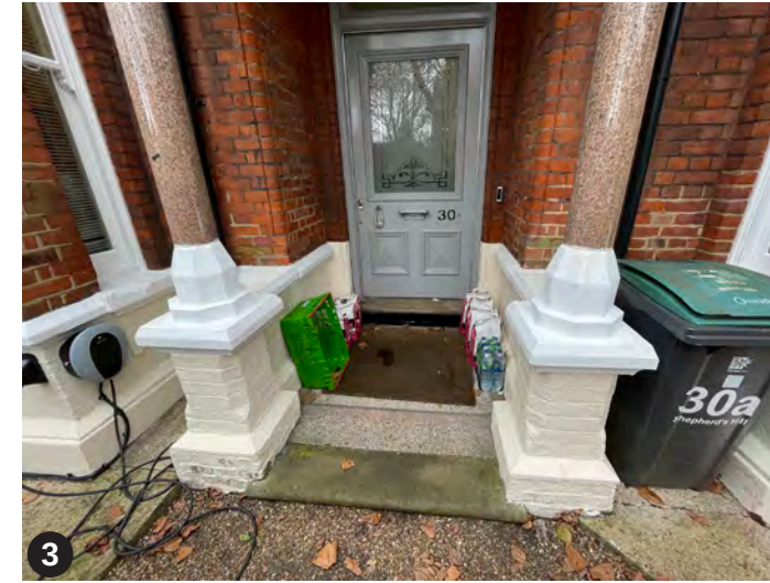
3 Entrance to 30 a ( Application Property)
