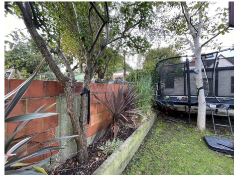
fig 6.4 Garden elevation of existing garage
