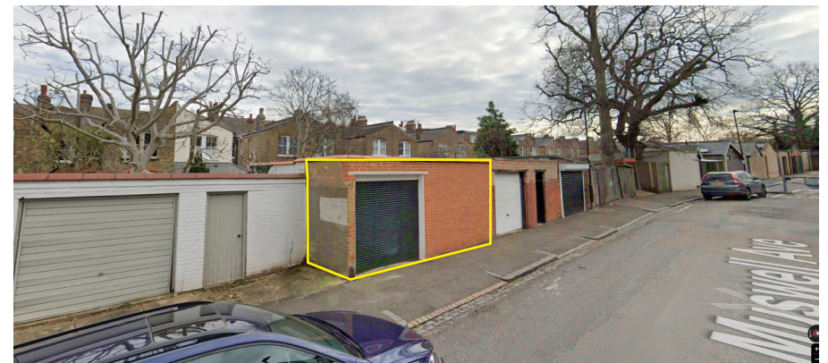
fig 2.2 Rear street view from Muswell Avenue showing site outlined in yellow
