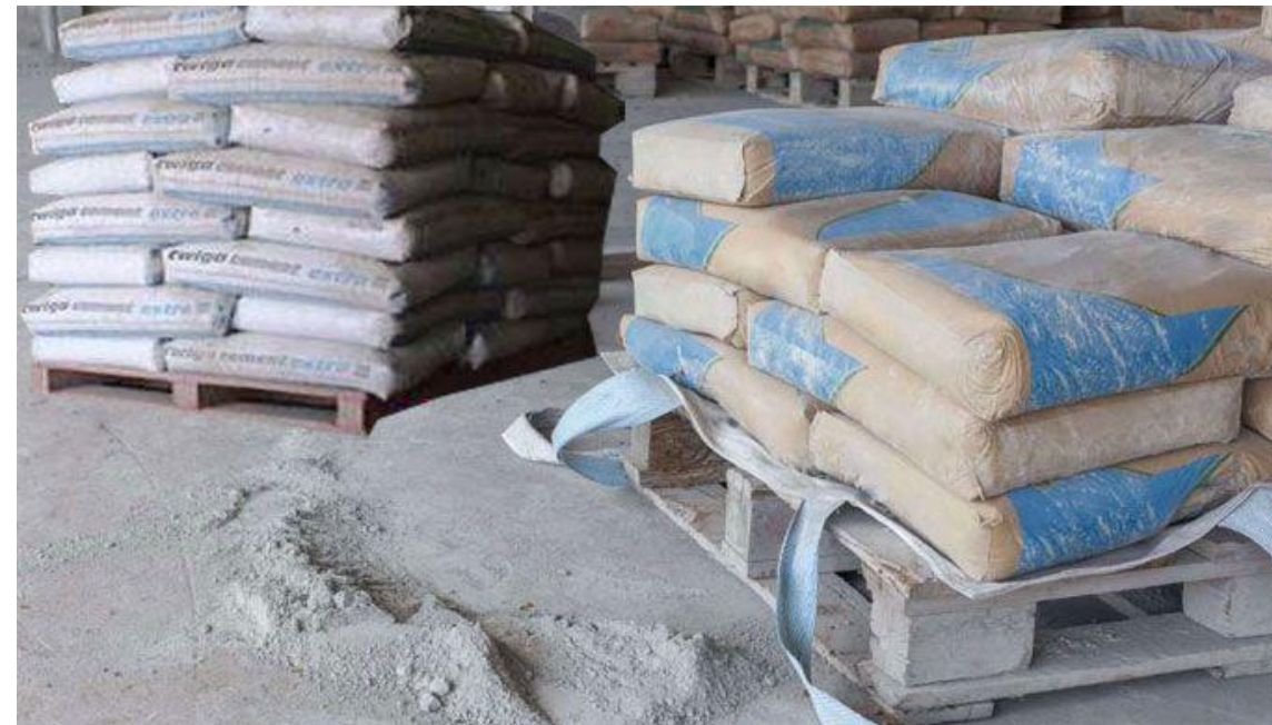
FIGURE 10 – EXAMPLE OF CEMENT STORAGE.
