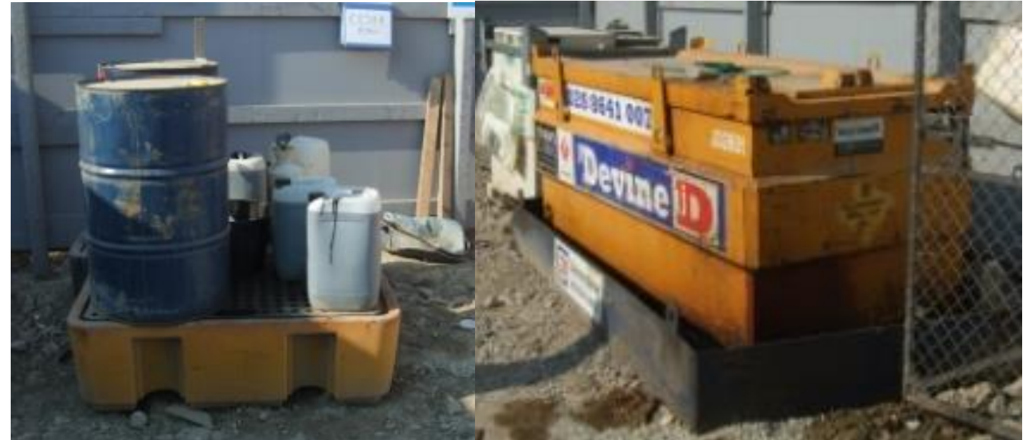
FIGURE 09 – EXAMPLE OF FUEL TANKS BUNDING.
