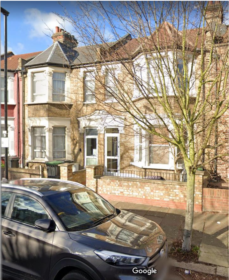
FIGURE 01– VIEW ELEVATION AT 89 WILLINGDON ROAD VIEW.
