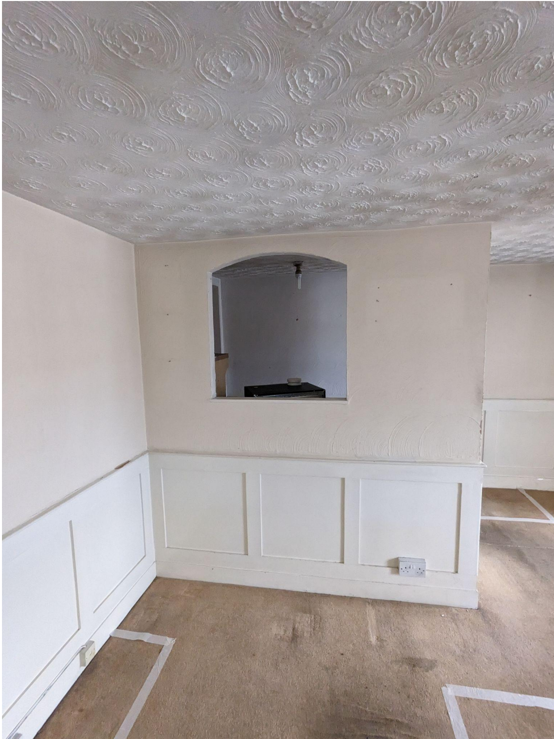
Internal view of wall proposed to be removed 1
