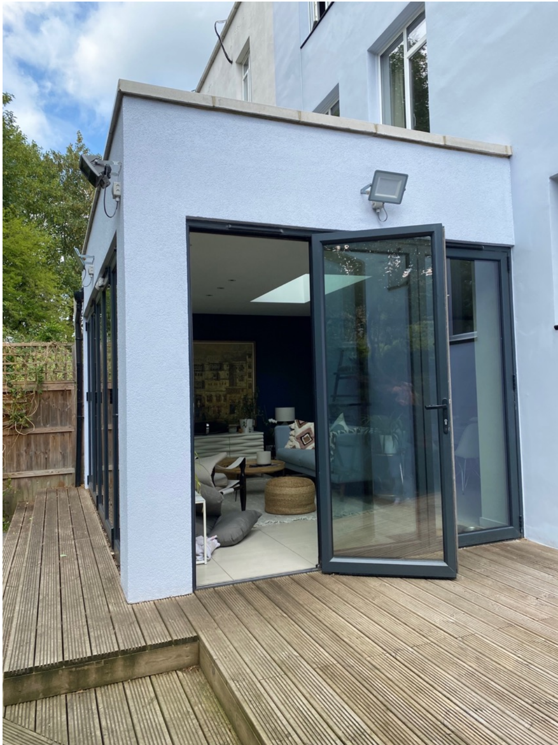
Existing rear extension view
