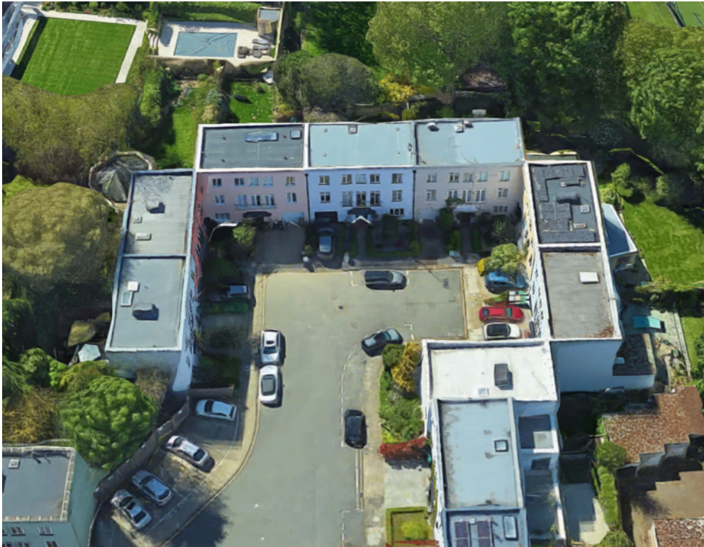
Front elevation aerial view
