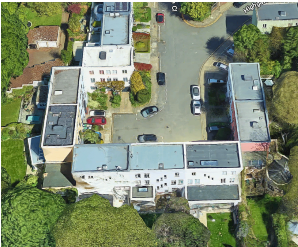
Rear elevation aerial view
