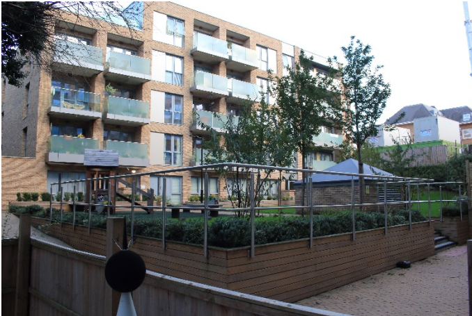
Location 1 looking west
