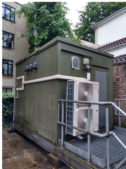
Figure 8-10: Examples of the telecoms equipment existing on the roof and at ground level
