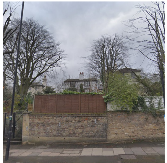
Figure 7: 50-54 North Hill, Grade II listed houses set back from the street
