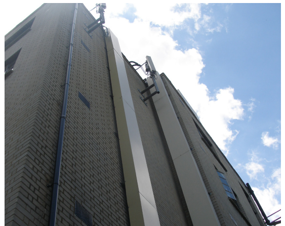
Figure 13: Example of the ducting and antennas attached to the side of the building
