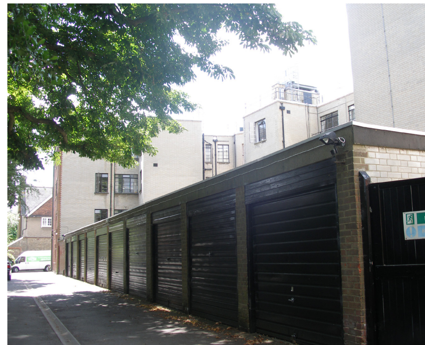
Figure 3 (top): Existing building. Figure 4 (bottom left): Unsightly telecommunications equipment to be removed. Figure 5 (bottom right): Existing garages to rear of the building.
