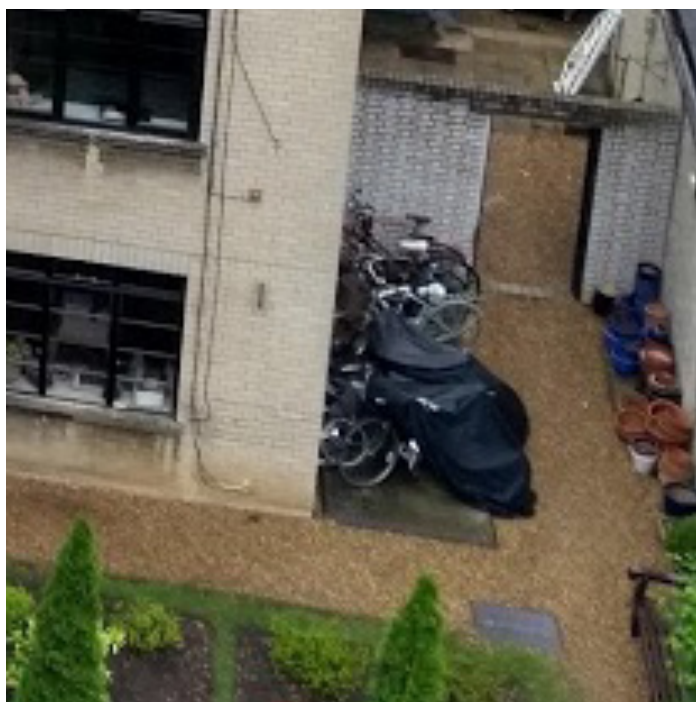
Figure 32 (top): Existing telecoms hut to be removed Figure 33 (bottom): Existing bicycle storage to be replaced and improved
