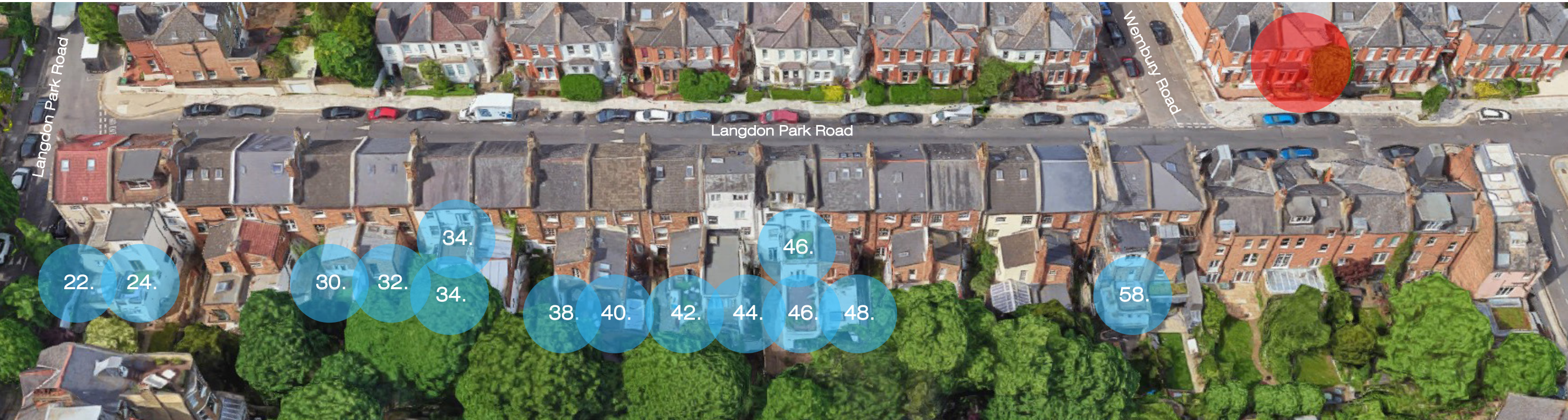
b. Roof Terraces on Langdon Park Road at numbers: 22, 24, 30, 32, 34 (2 roof terraces), 38, 40, 42, 44, 46 (2 roof terraces), 48 and 58.
