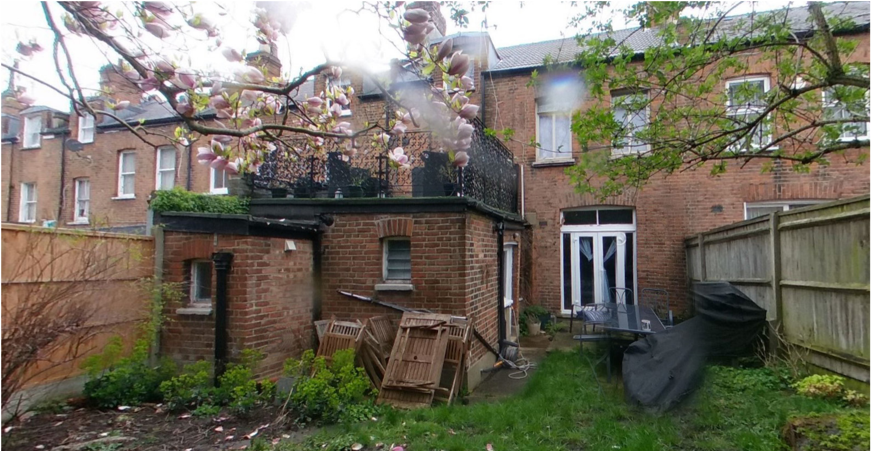
View north-east of existing rear extension and roof terrace at application site, 43 Langdon Park Road.
