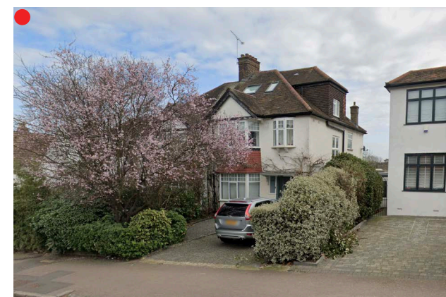
22 Coppetts Road (Application Site)
