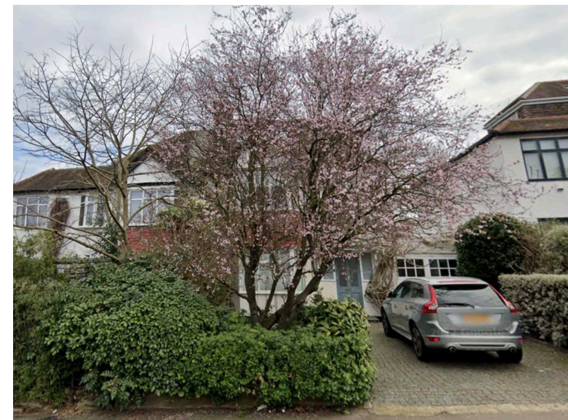
Existing street view of application site
