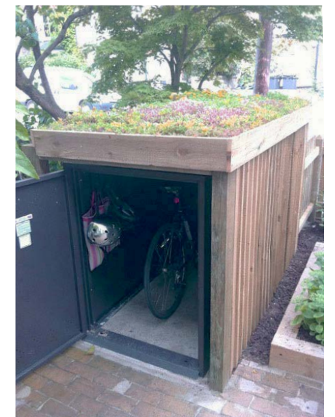
Bespoke clad bike locker w. green roof
