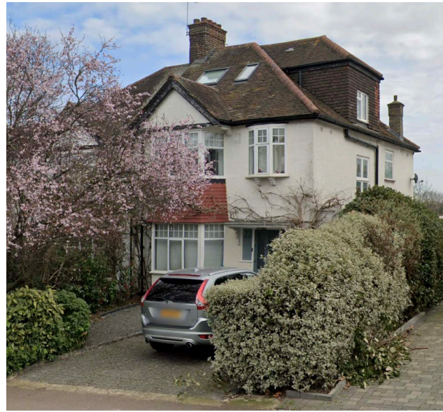
Existing Street View
