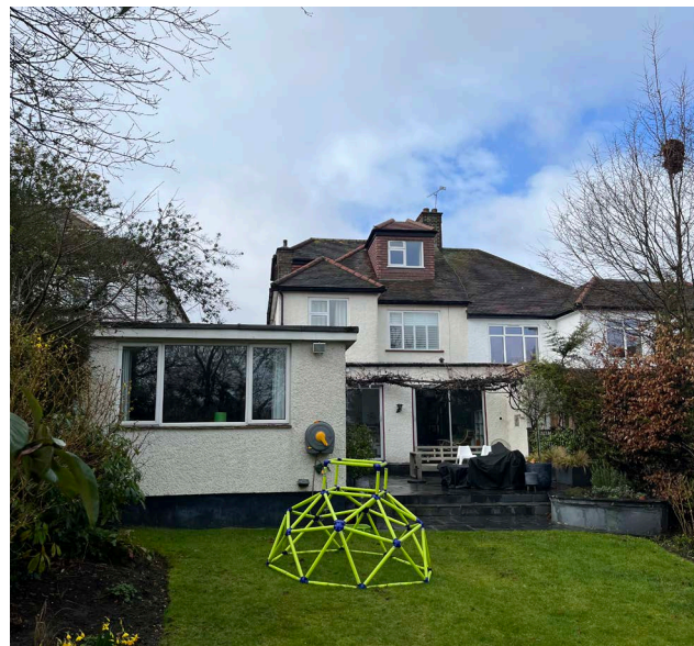
Existing Rear View
