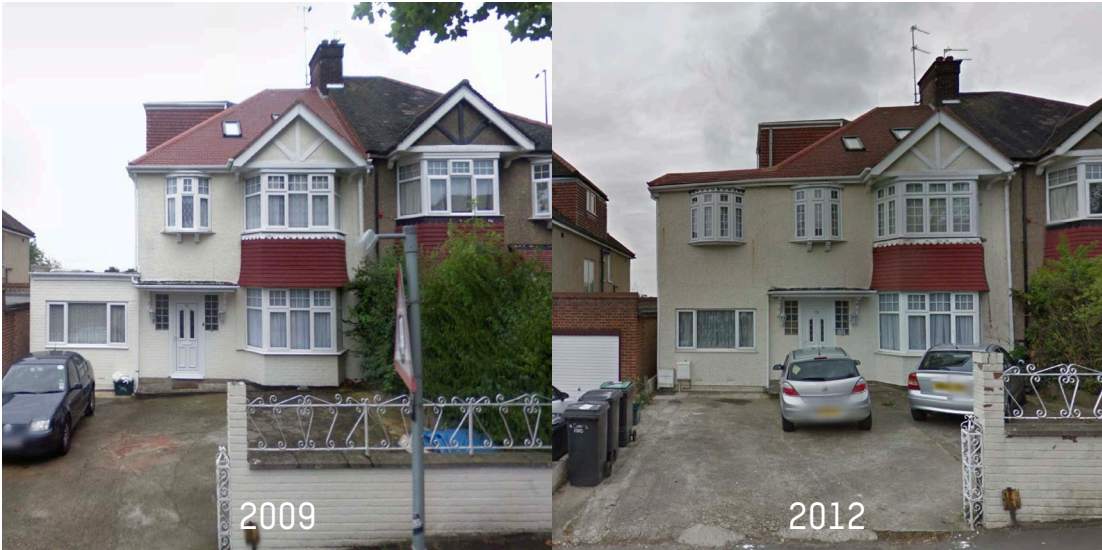
16 Coppetts Road: Google Street View
