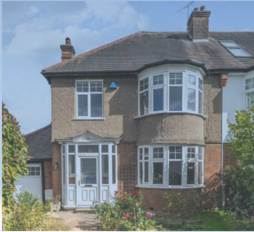
PHOTO OF THE EXISTING FORDINGTON ROAD ELEVATION
