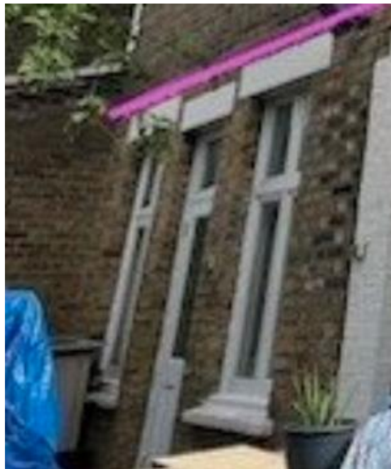
Front Elevation Ground Floor Windows
