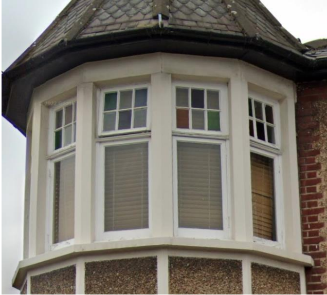
Front Elevation First Floor Window (South)
