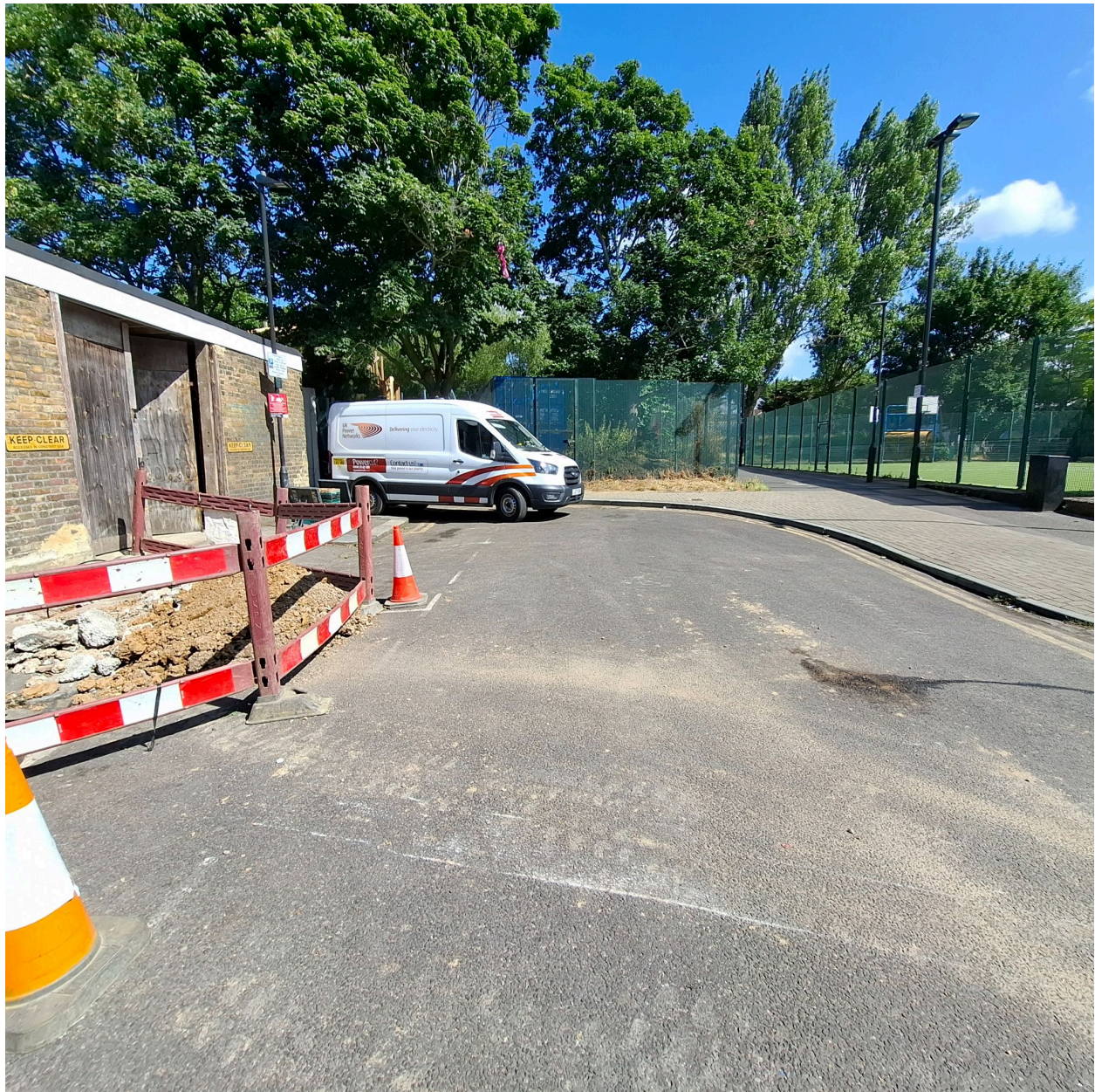
Fig 12. Towards end of Somerford Grove. (taken in Sept 2025)
