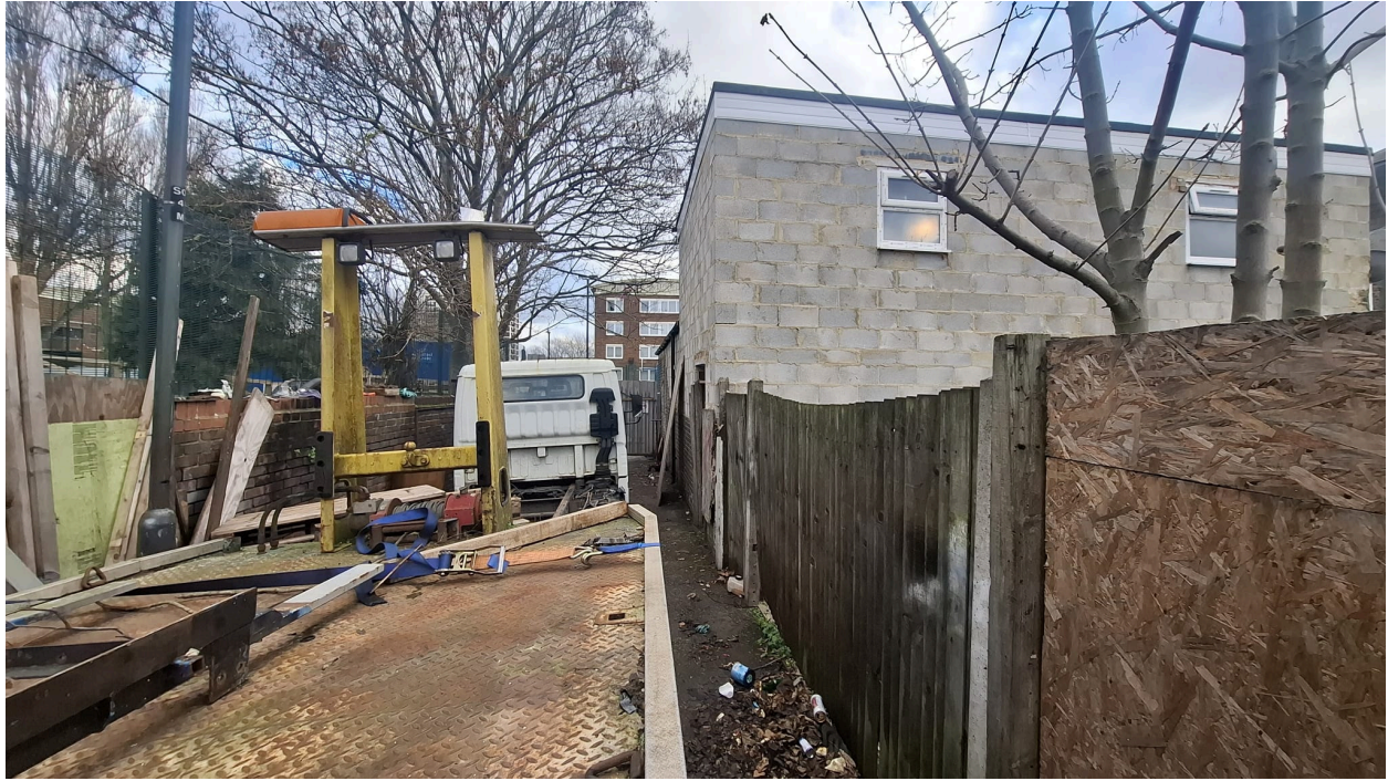
Fig 9 From North West.
