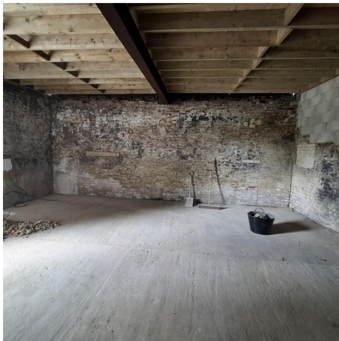
Internal condition of property with new roof structure
