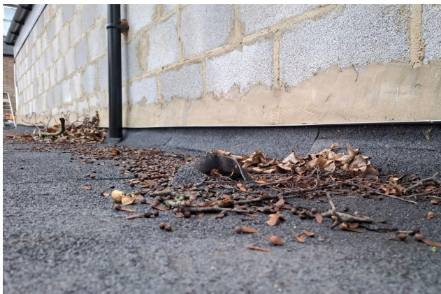
Leaves and twigs on lower flat roof.
