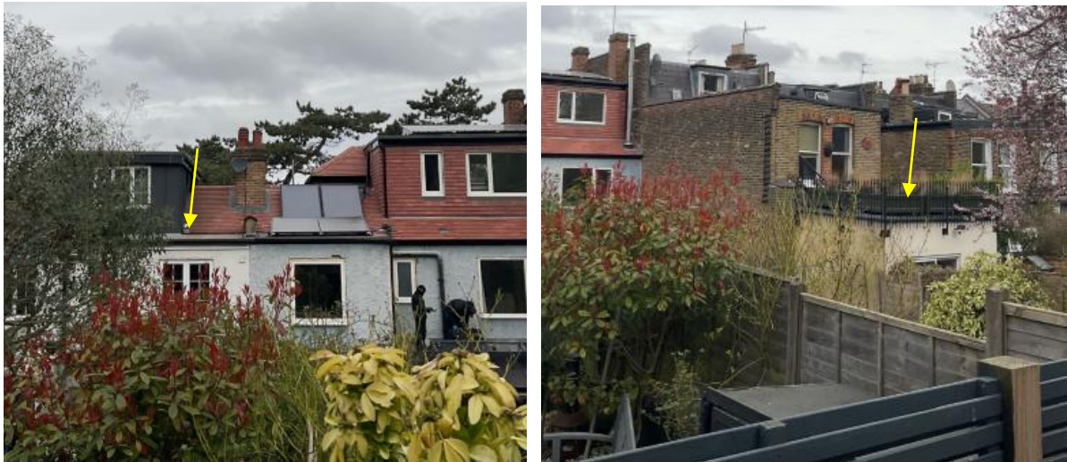
Rear view of the back of the terraces and existing railing and terrace to no 302.
