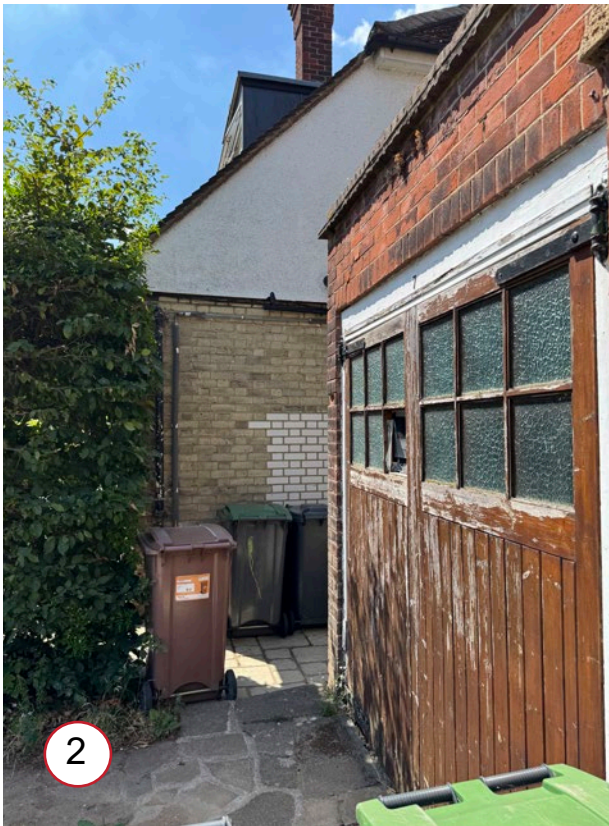
GARAGE DOORS AND SITE BOUNDARY
