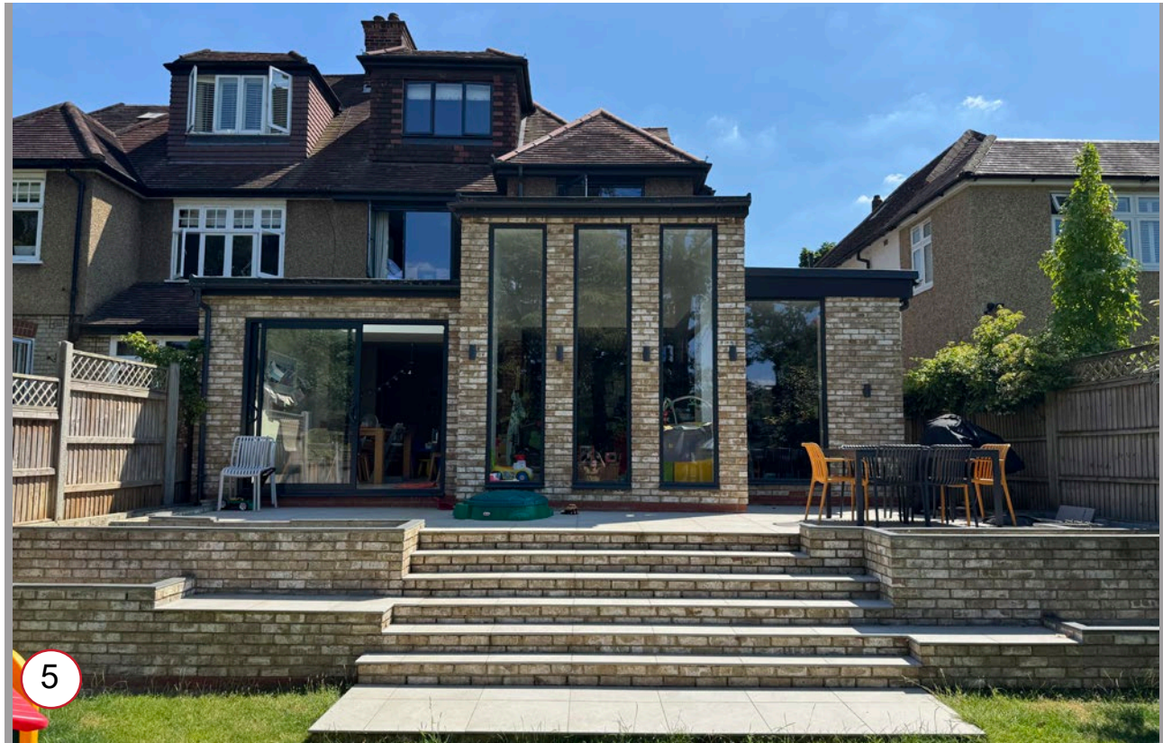
VIEW OF REAR
