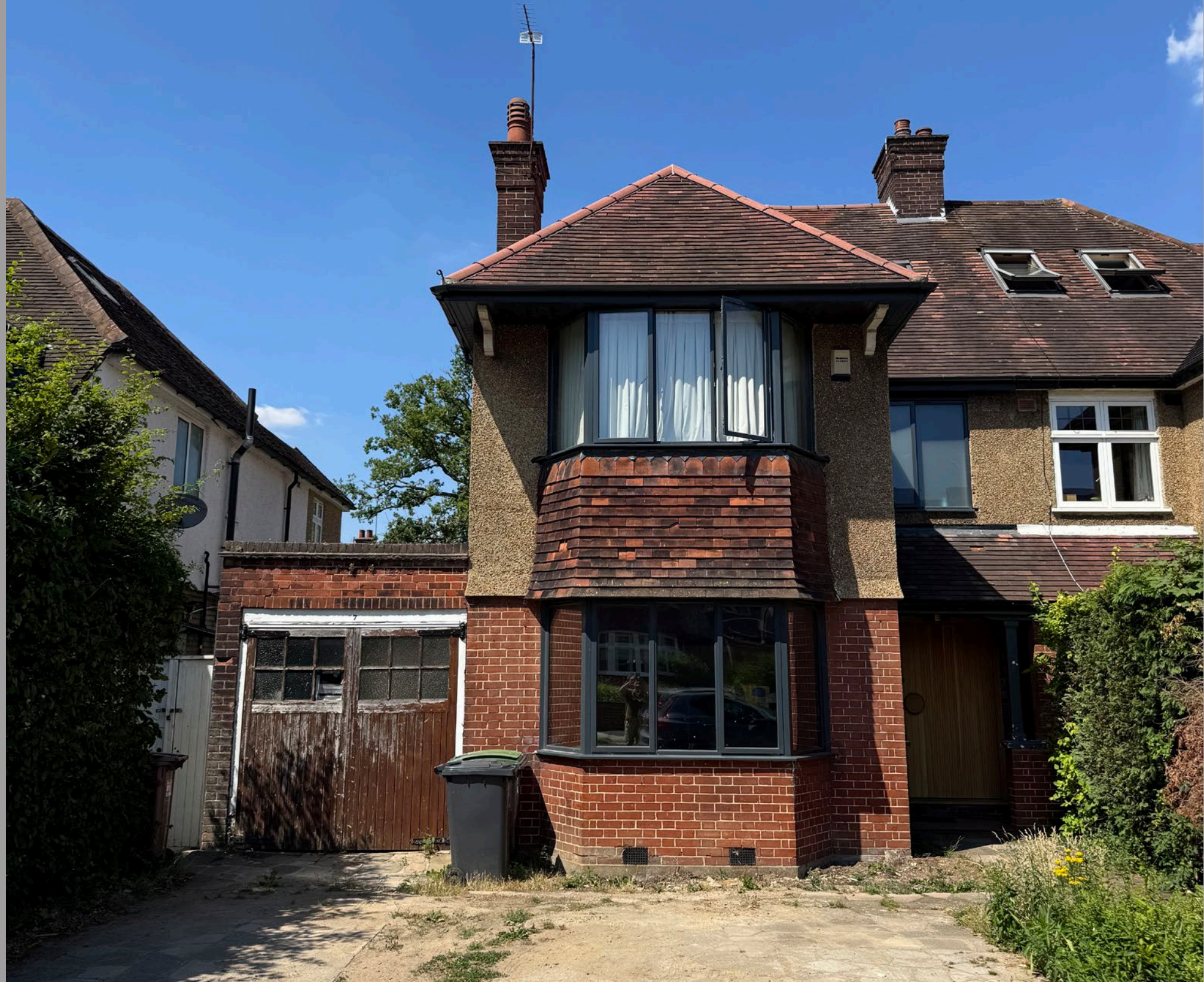
VIEW OF EXISTING HOUSE LOOKING NORTH FROM TWYFORD AVENUE
