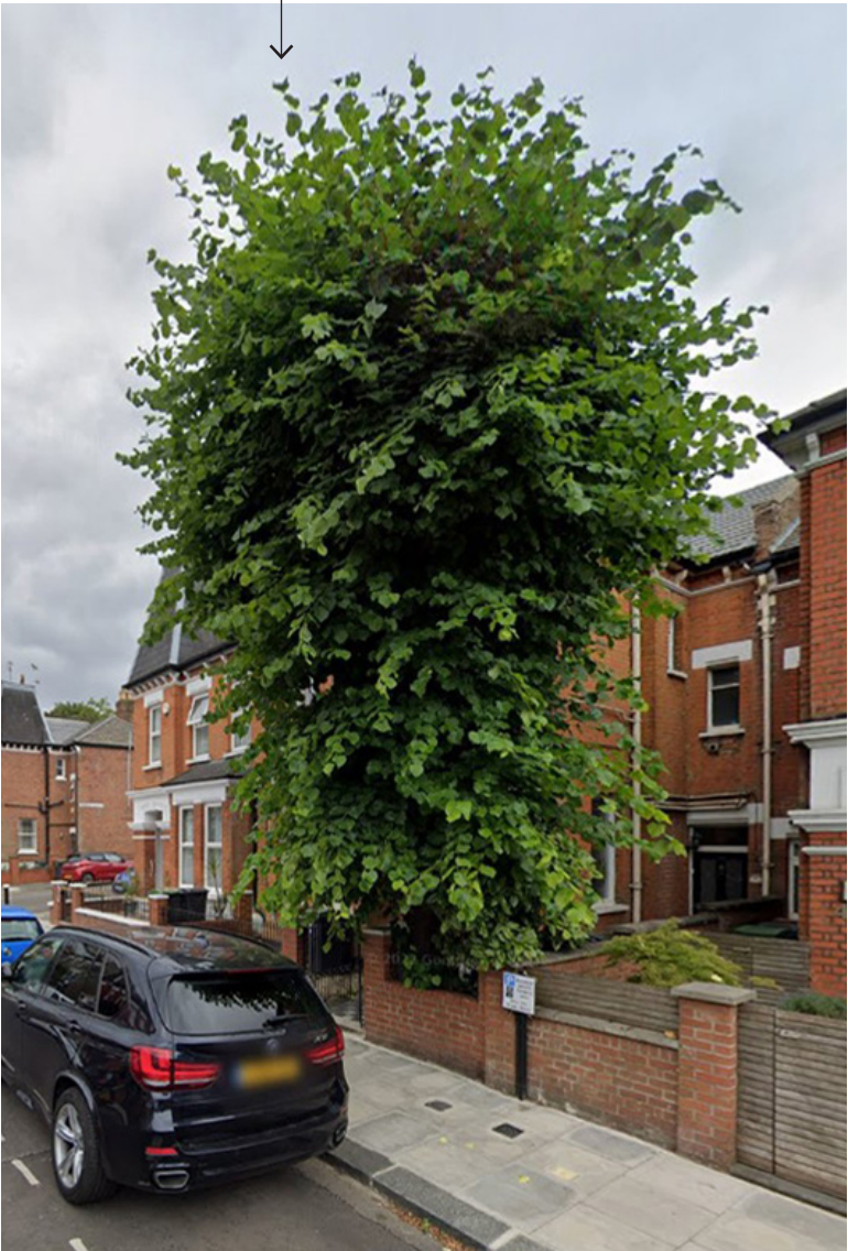
View south of 43 Langdon Park Road front and adjoining garden of 45 Langdon Park Road. Lime tree sited 2.4m from front of property.
