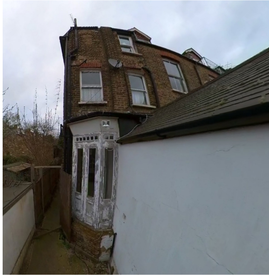
Fig 8. Existing non-original extension
