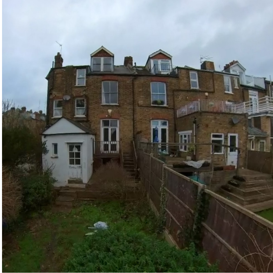
Fig 7. Existing rear condition photo
