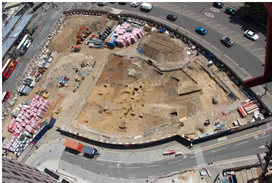
Plate 10: The Site Looking south
