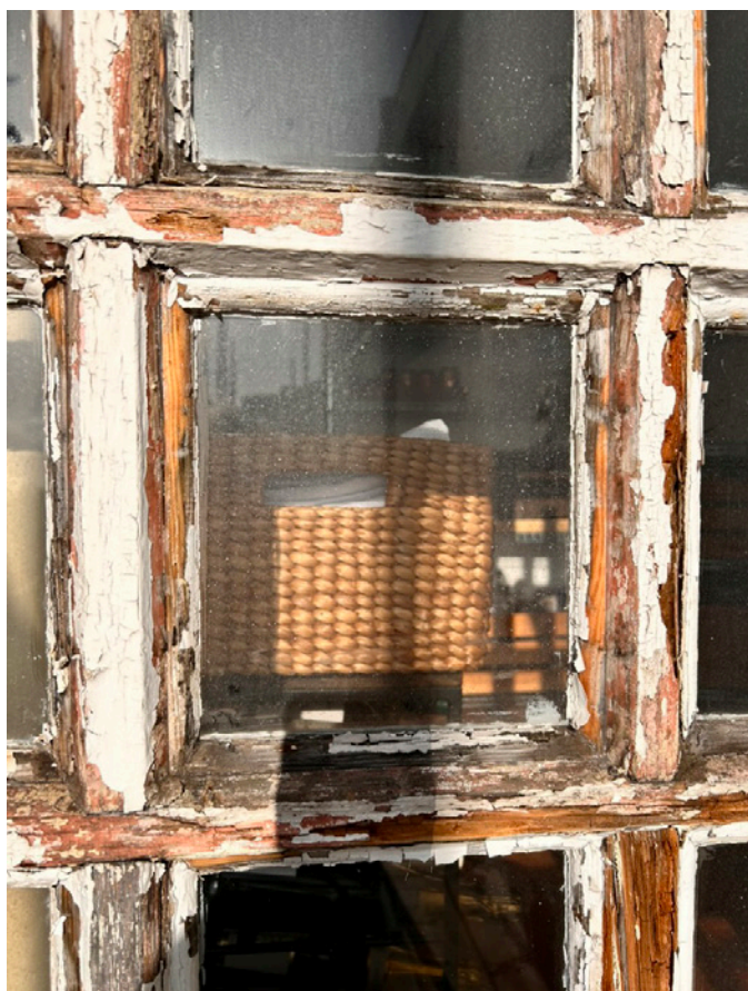
Loggia window photos - showing extent of rotten timber as revealed following paintwork being stripped
