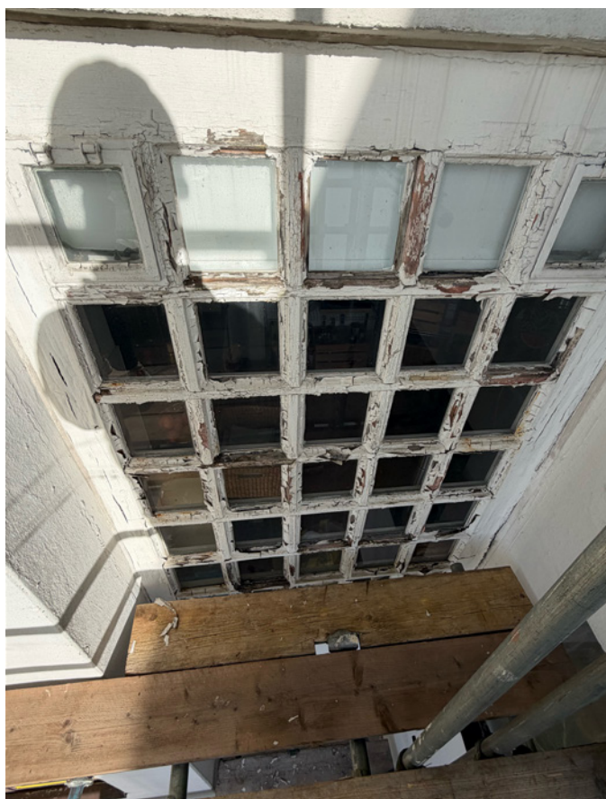
Loggia window - prior to paintwork being stripped
