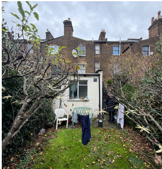
Figure 2: Photo of existing rear
