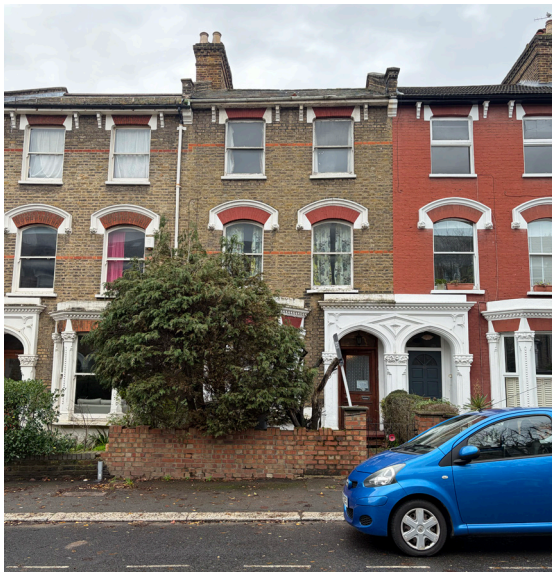
Figure 1: Photo of existing frontage
