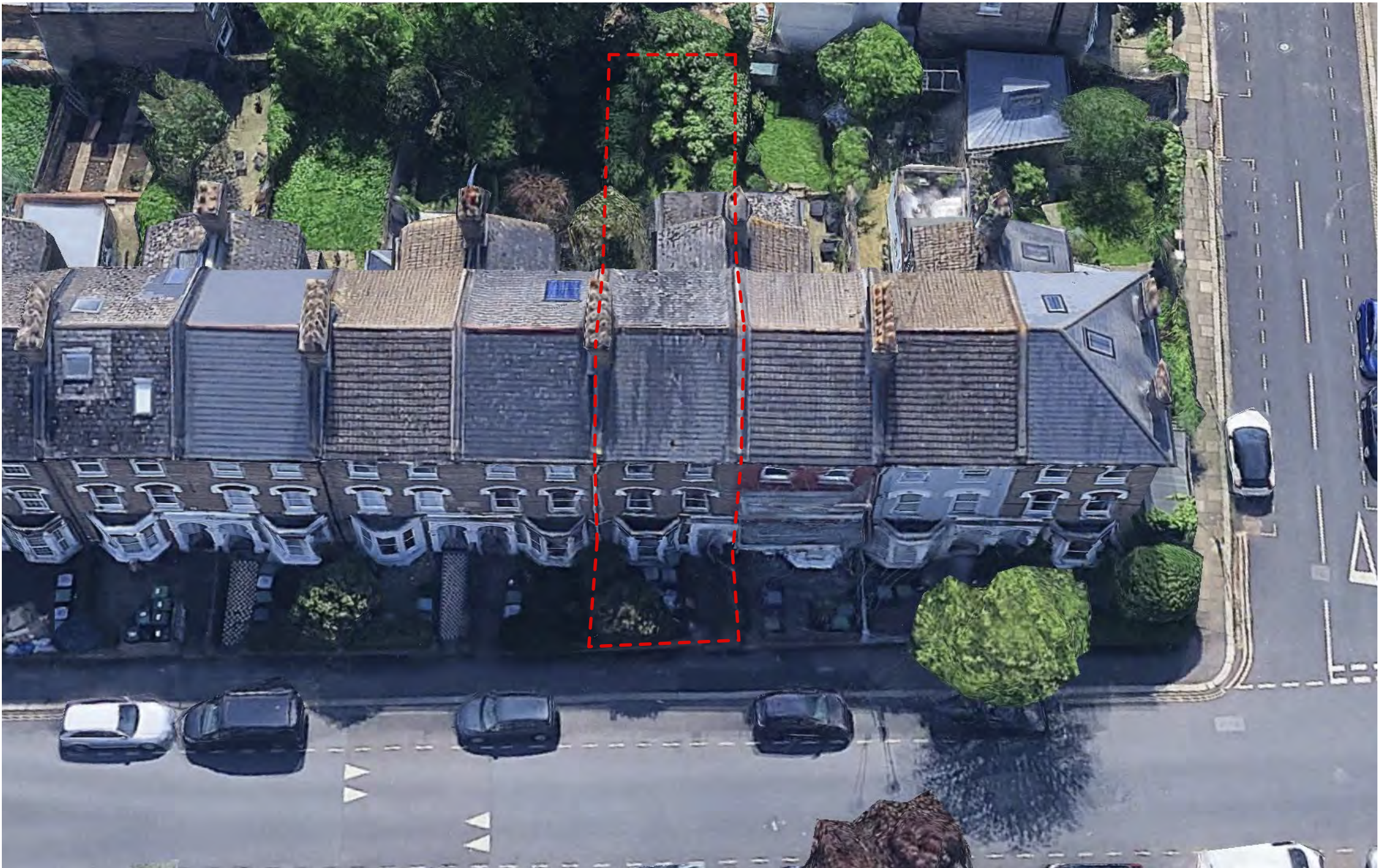
4: Site overview from North - in context of existing streetscape along Florence Road.
