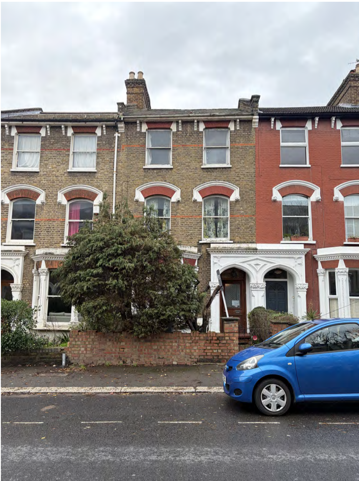
1: Existing photo of frontage to 80 Florence Road
