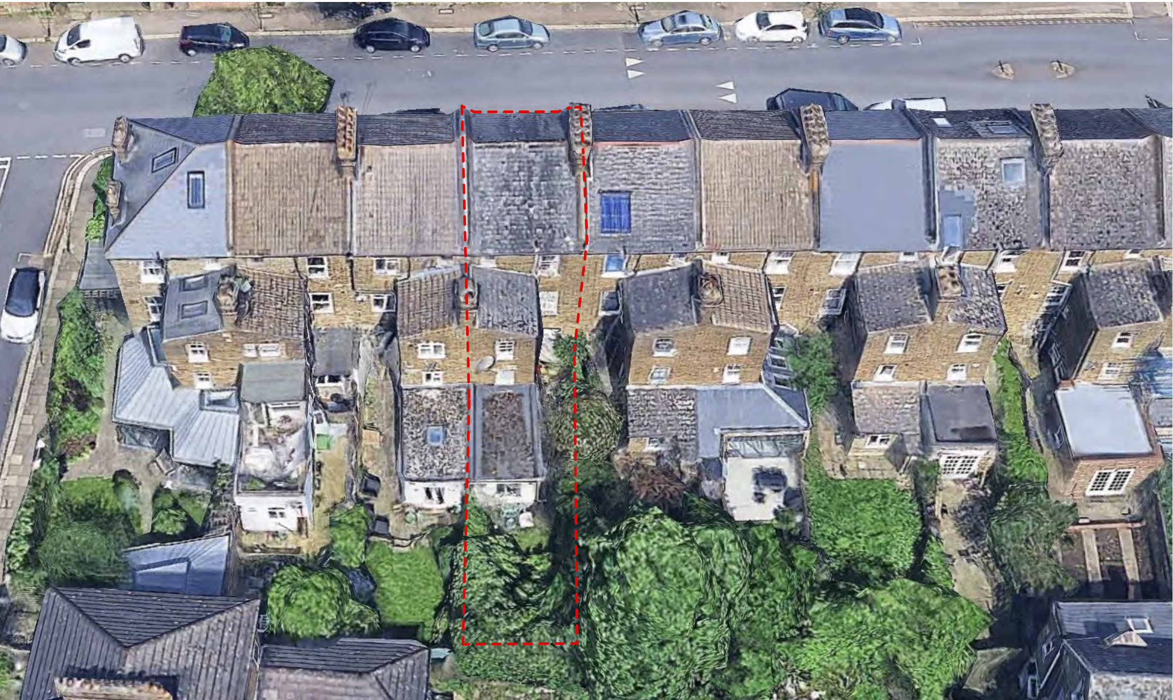
5: Site overview from South - in context of existing rear extensions on Florence Road.
