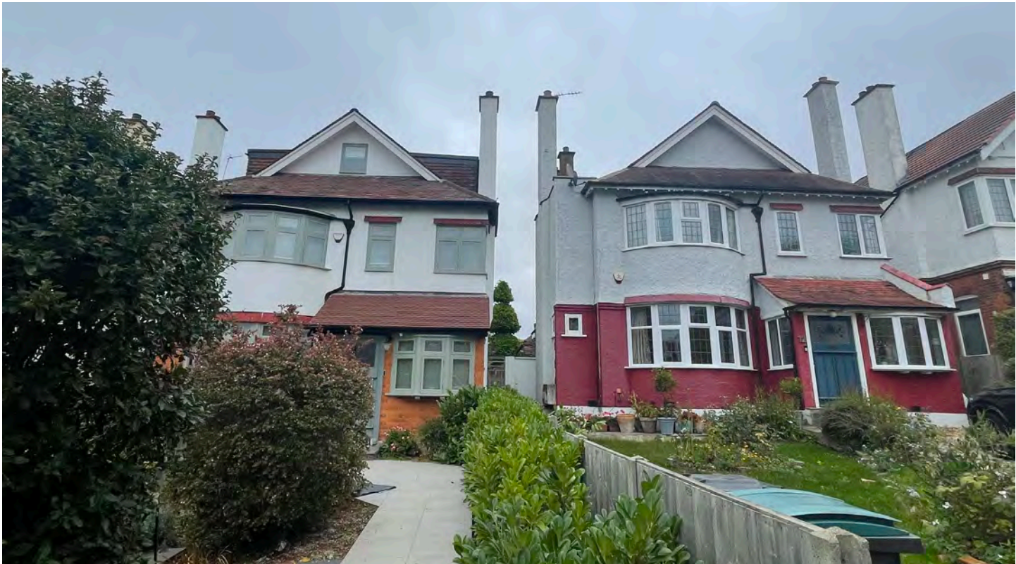
Figure 19: Existing View between 14 & 12 The Avenue front facade
