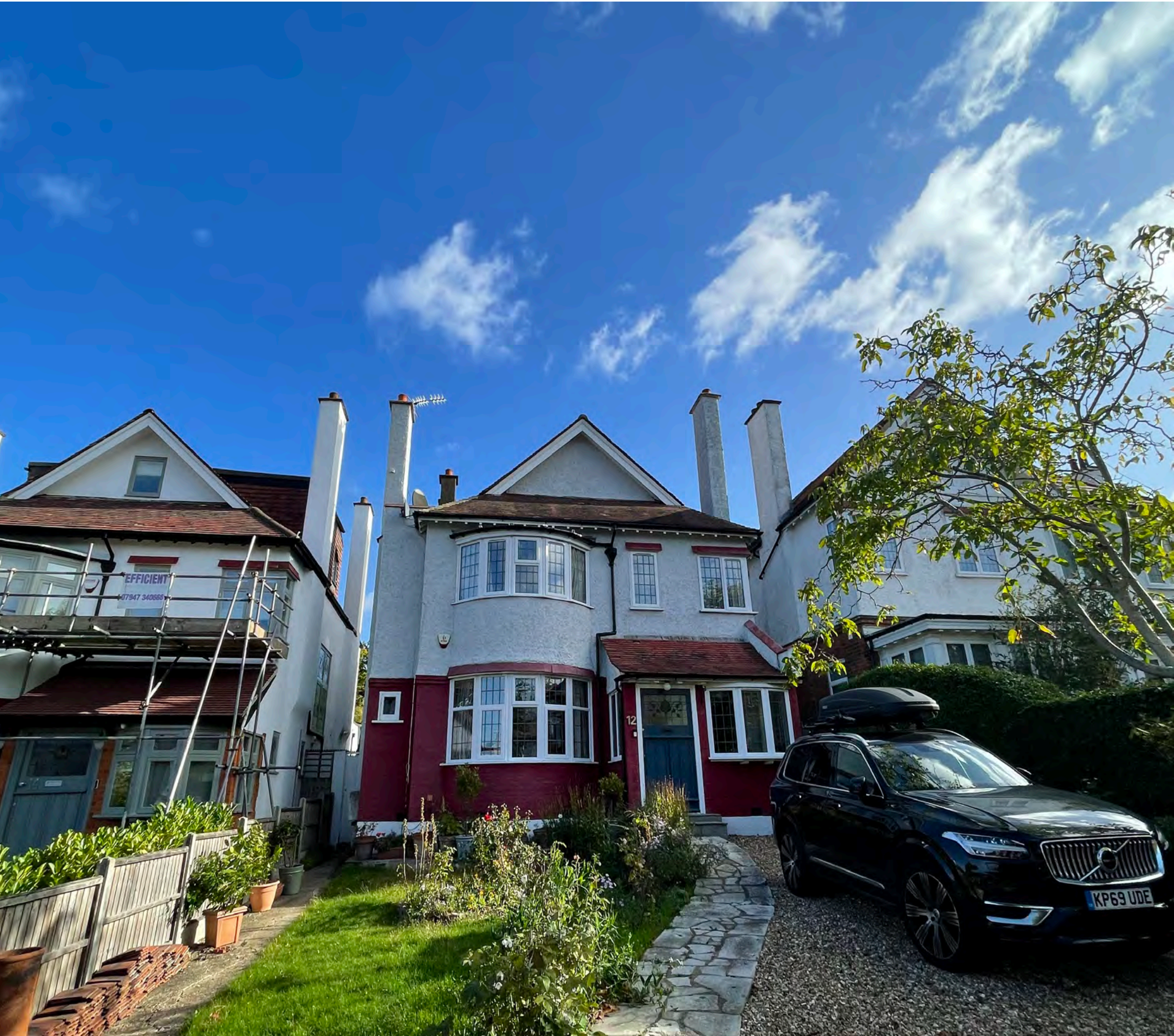
Figure 1: Site location and wider street context of 12 The Avenue within the Vallance Road Conservation Area
