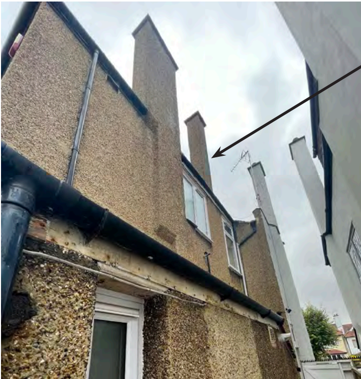
Figure 18: Chimney stack to be removed
