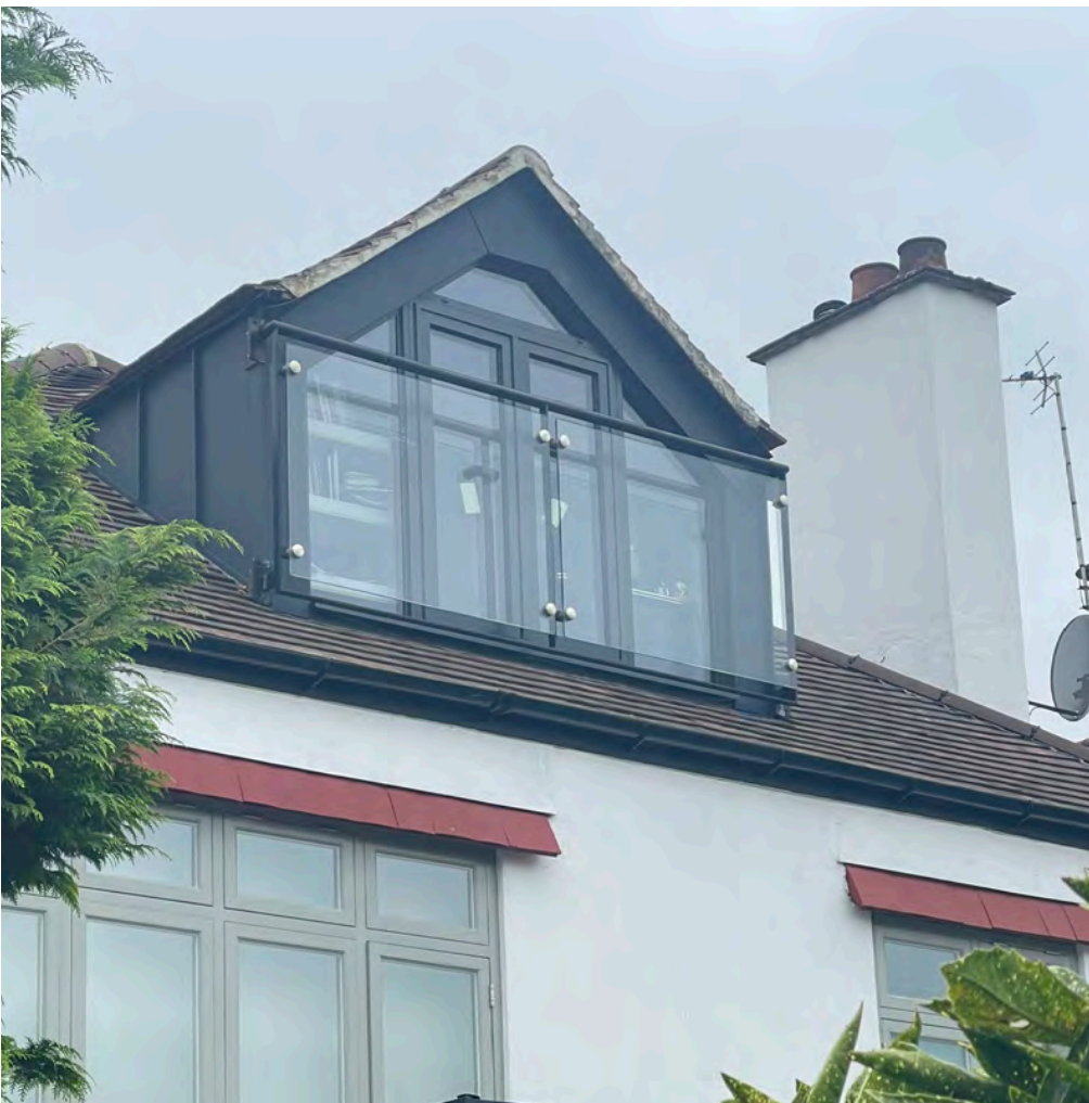
Figure 10: Rear View of Existing gable dormer extension at 14 The Avenue
