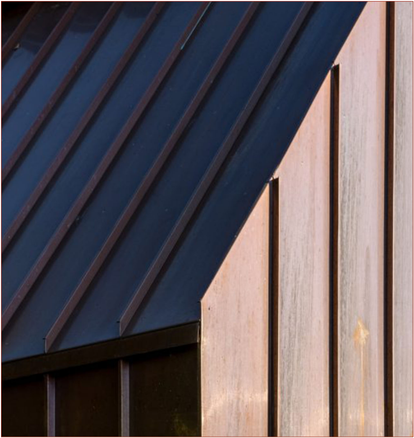
Dormer clad in supplier VMZINC standing-seam zinc colour pigmento (Referential image- not to scale)
