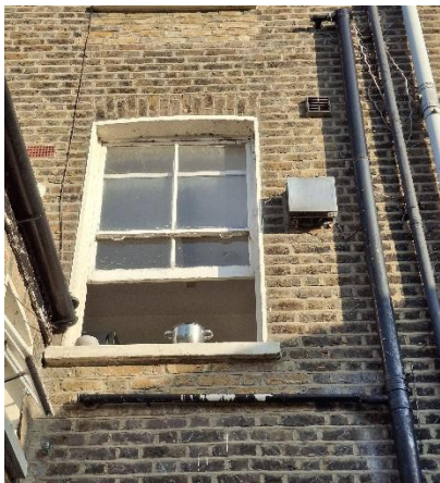
Rear elevation – Timber sash window (First floor)
