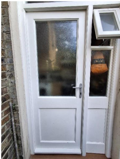
Rear elevation – Timber exit door with adjoining top hung window to the right. (Ground floor)
