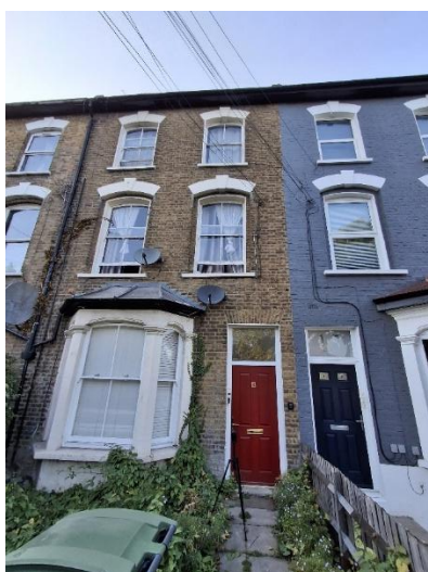
Front Elevation of 13 White Hart Lane
