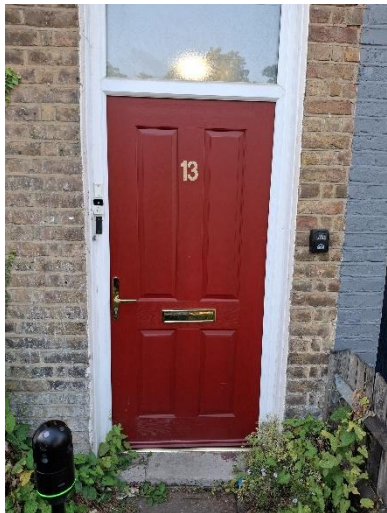
Front elevation – Timber front entrance door (Ground floor)
