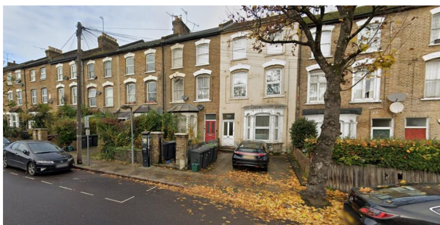
The Site viewed from a distance – Front elevation (Property with Red door)
