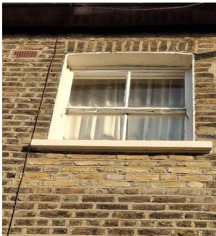
Rear elevation – Timber sash window (Second floor)
