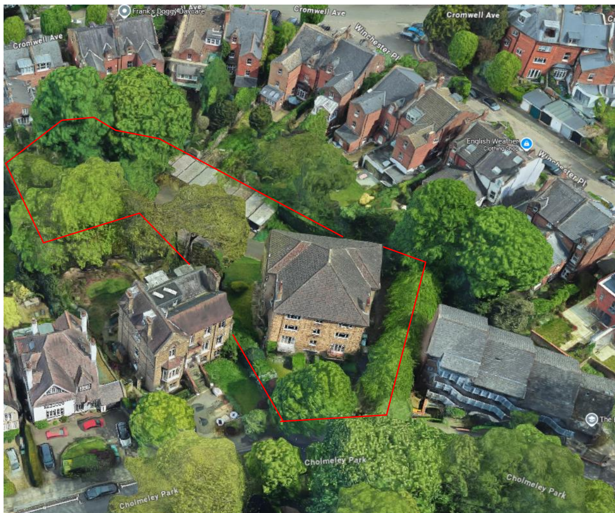
Figure 1: Aerial view of site from the west with indicative red line boundary
