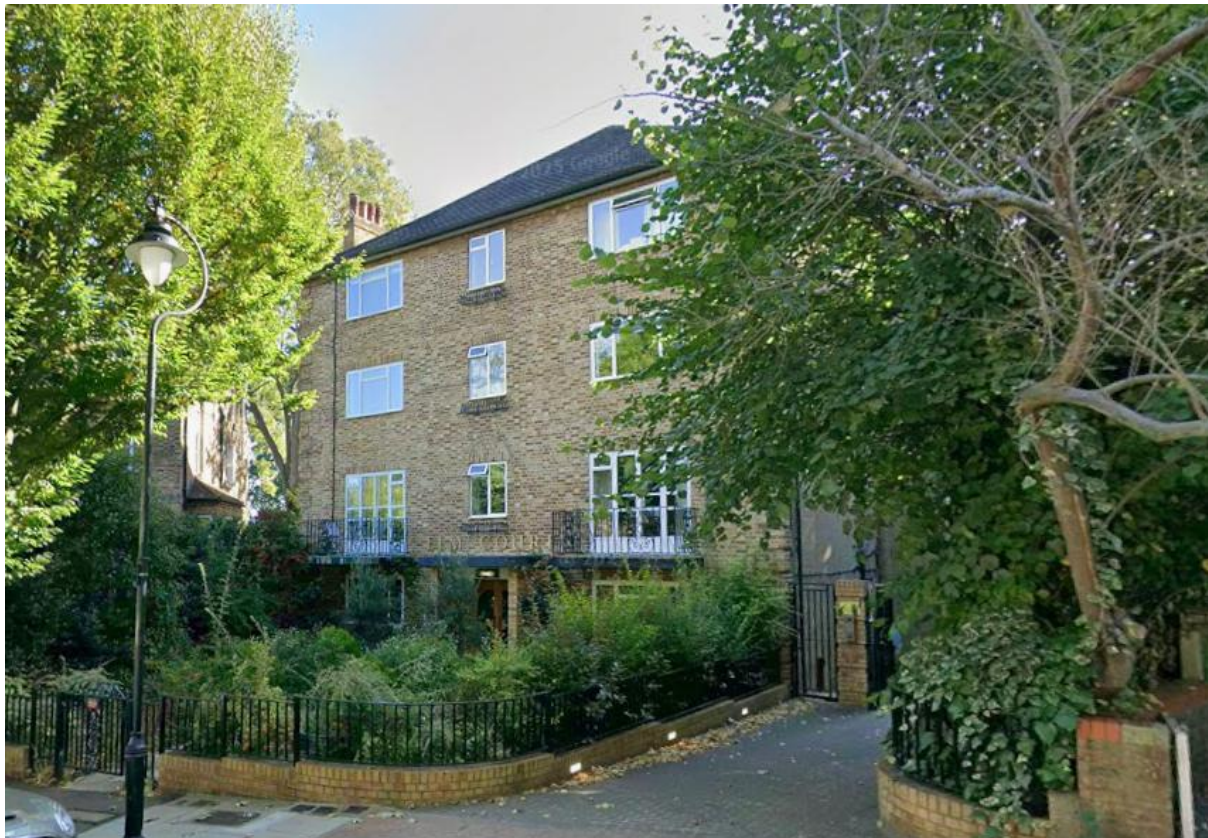
Figure 1 – Street View of Site
