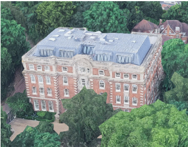
Figure 15 Furnival House showing mansard roof.
