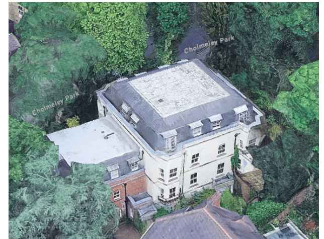
Figure 17 Flats opposite the site showing mansard roof construction.
