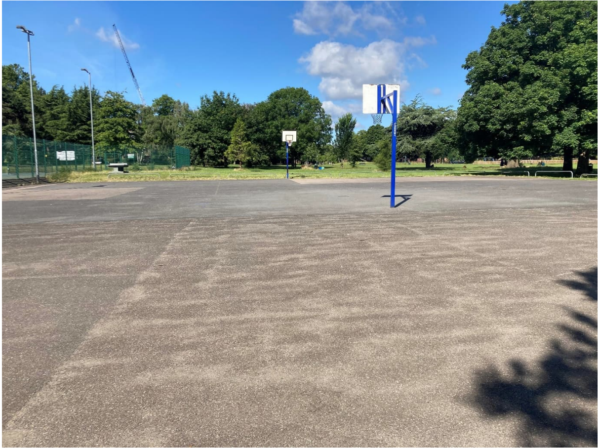
View of the existing location
