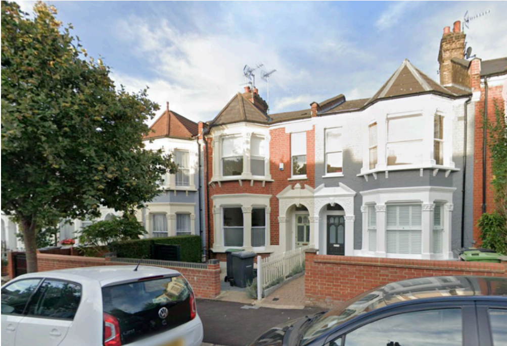
Front view of property from the street
