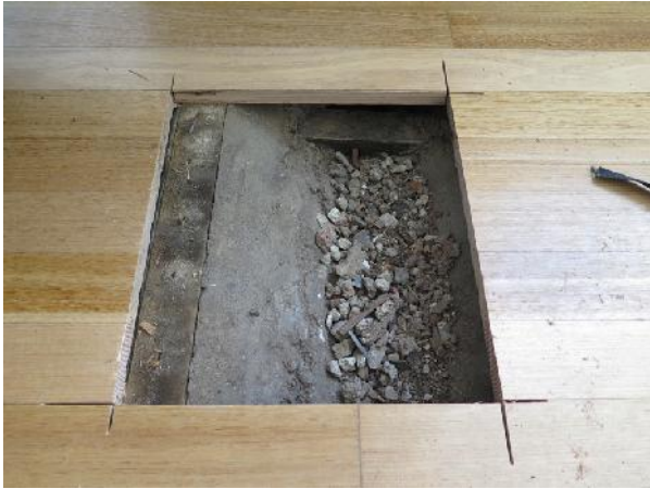
Photos of the flooring substrate taken during 2014 works. This material was removed as per the approved demolition to reveal brick and rubble beneath.
