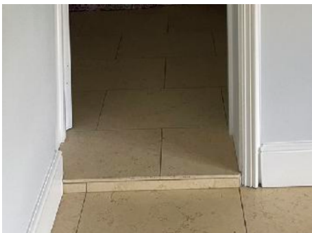
Slight level change into store room
