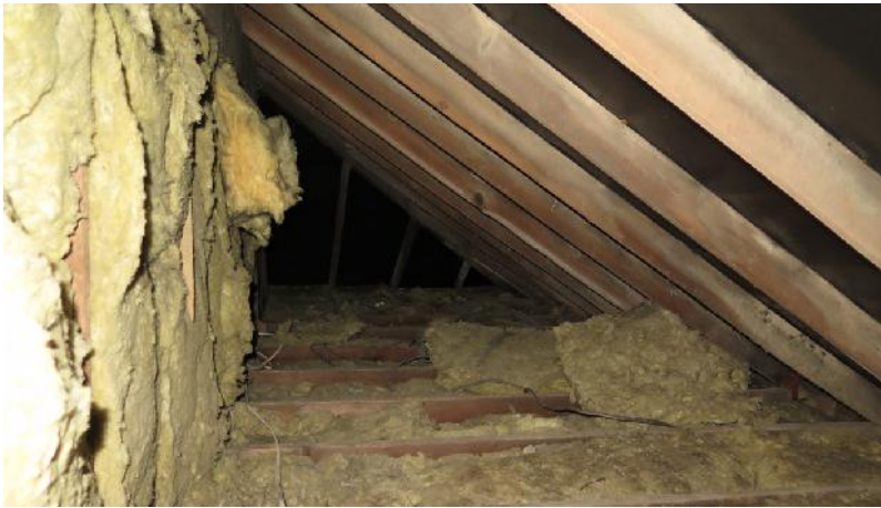
Photos of the existing roof structure
