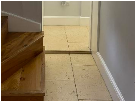
Slight level change into WC
