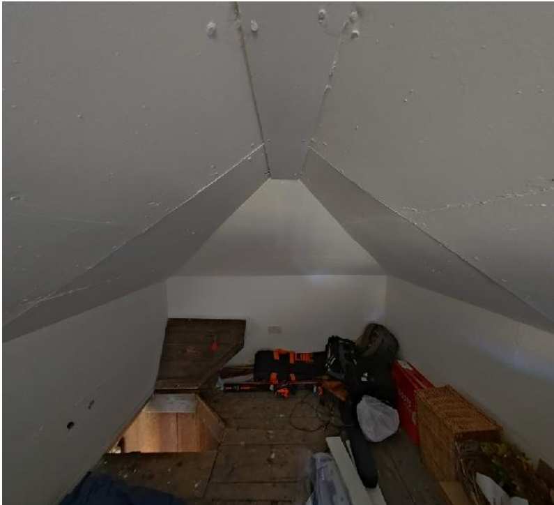
Photos of the attic space from 2025
