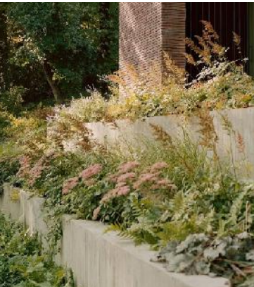
Textured retaining wall
