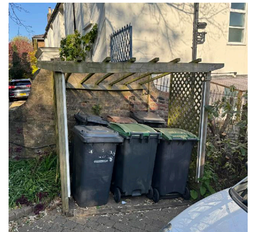
Existing bin store
