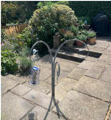
Existing external stairs to be reconfigured
