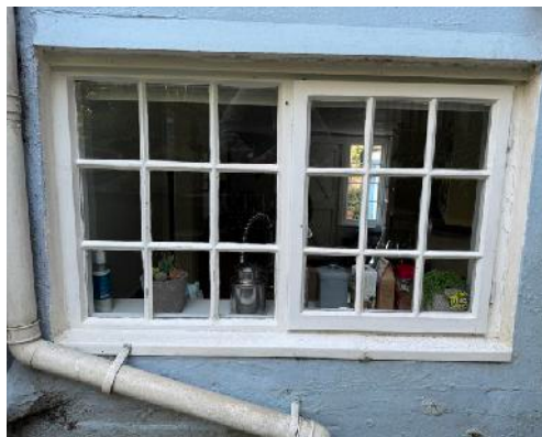
WT-3 9 pane side casement and fixed casement
