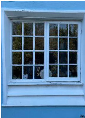
WT-5 12 pane side casement and fixed casement
