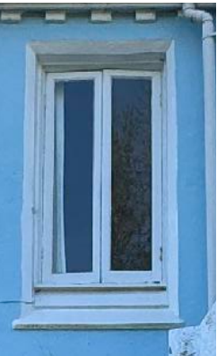
WT-8 1 pane horizontal pivot casement
