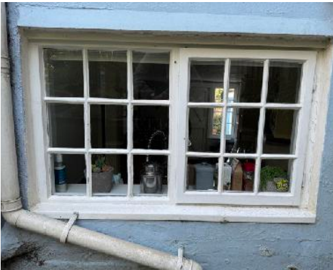
WT-3 9 pane side casement and fixed casement
