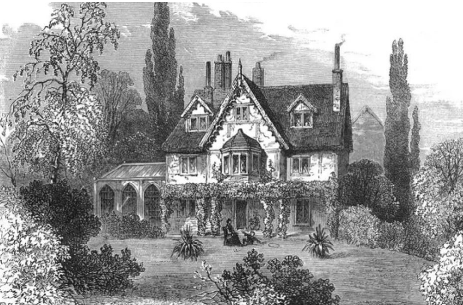
Ivy Cottage (image: 1825) Highgate, London, built 1819, demolished in 1934
