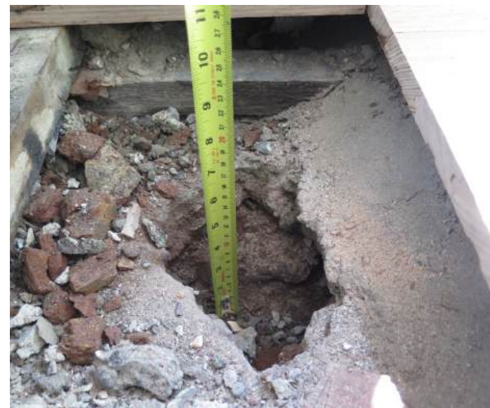
Lower ground floor opening up to reveal floor buildup
