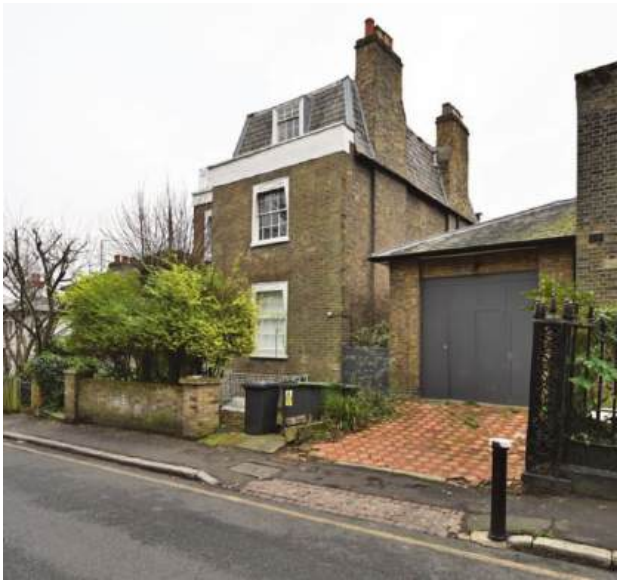
12 Wood Lane, Grade II listed (1816-41)
