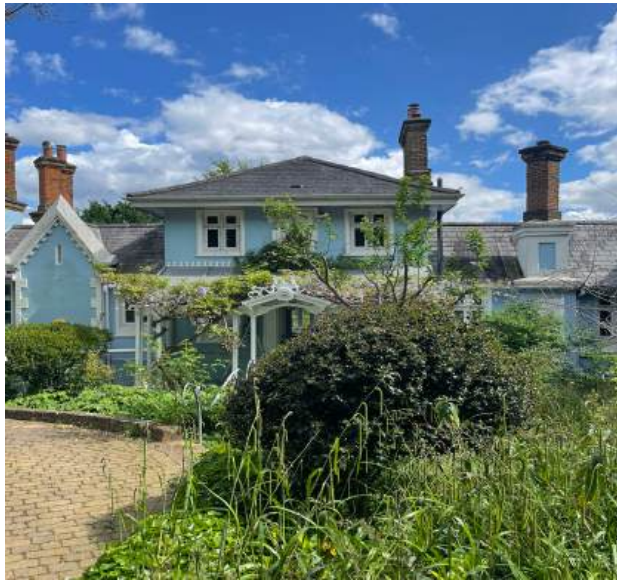
28 Wood Lane, Grade II Listed (1830's)
