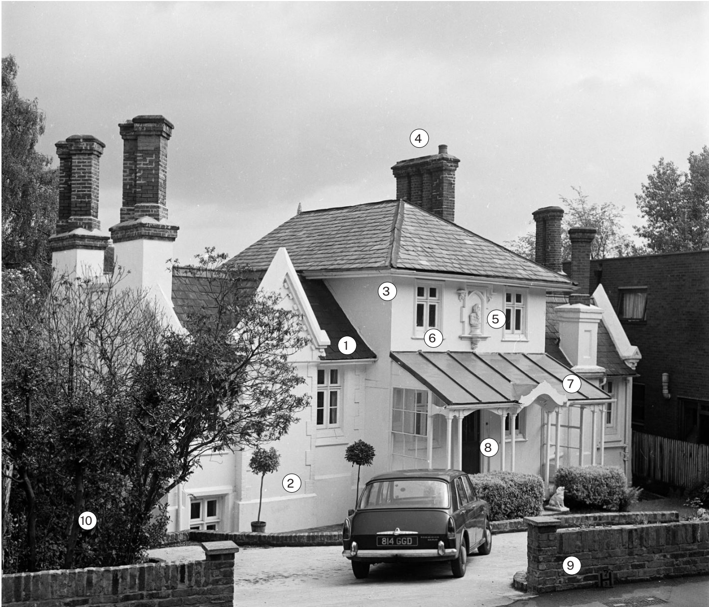
28 Wood Lane street front elevation, image c.1969-1974 Historic England
