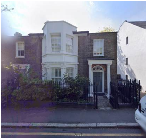
10 Wood Lane, Grade II listed (1830's)
