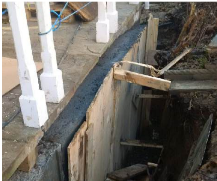
Trench excavation around porch -damp repair works
