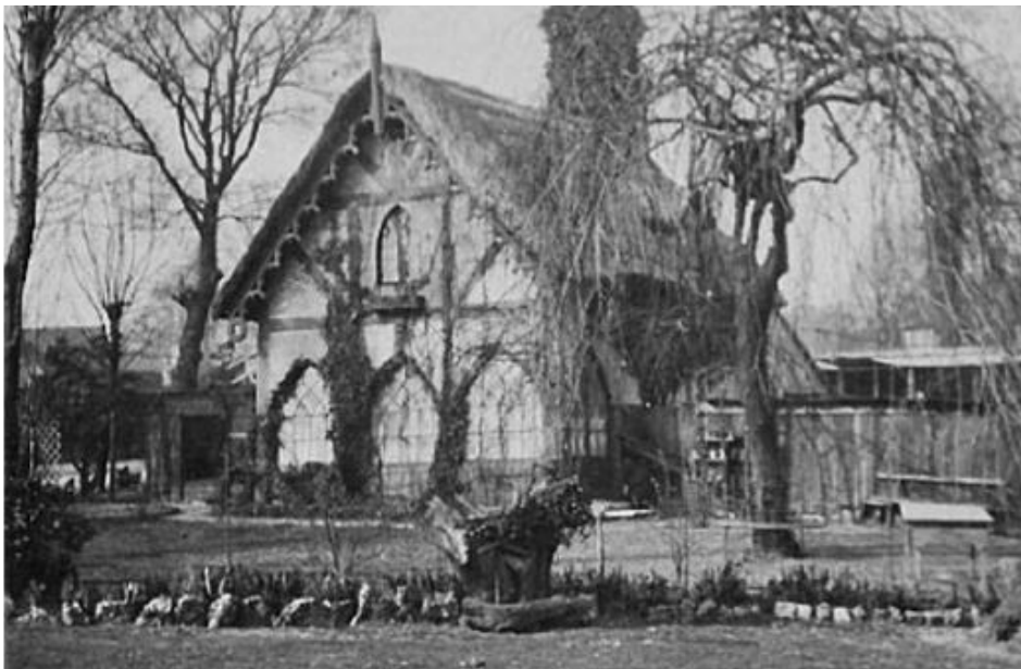
Fitzroy Farm Cottage (Photo. 1907)
