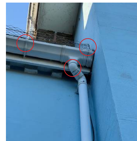
Series of images identifying external alterations to building fabric, including pipework, guttering, fascia boards and additional services
