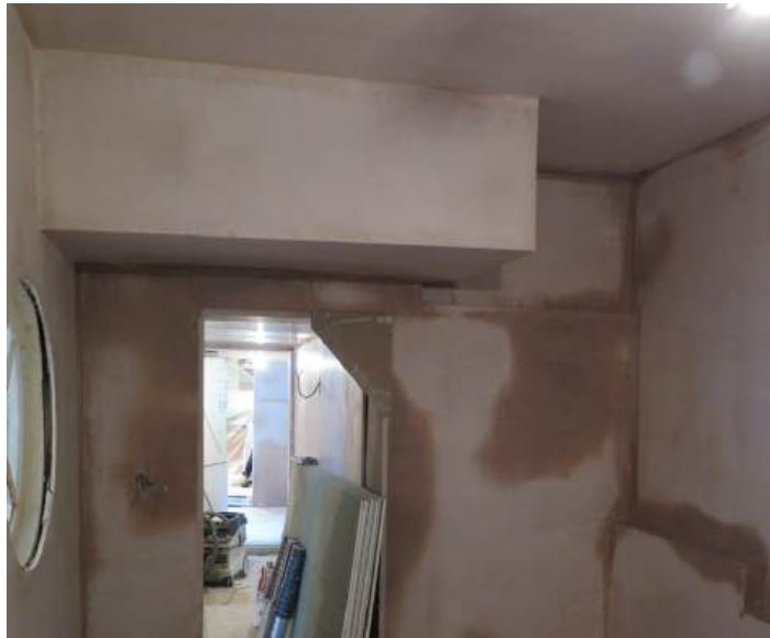
Lower ground floor east - bulkhead formed by remnant winders over
