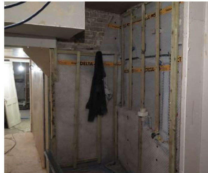
Lower ground northeast-drained cavity installation
