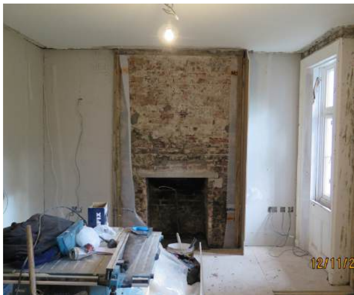
Lower ground floor east reception-mouldings to be reinstated
