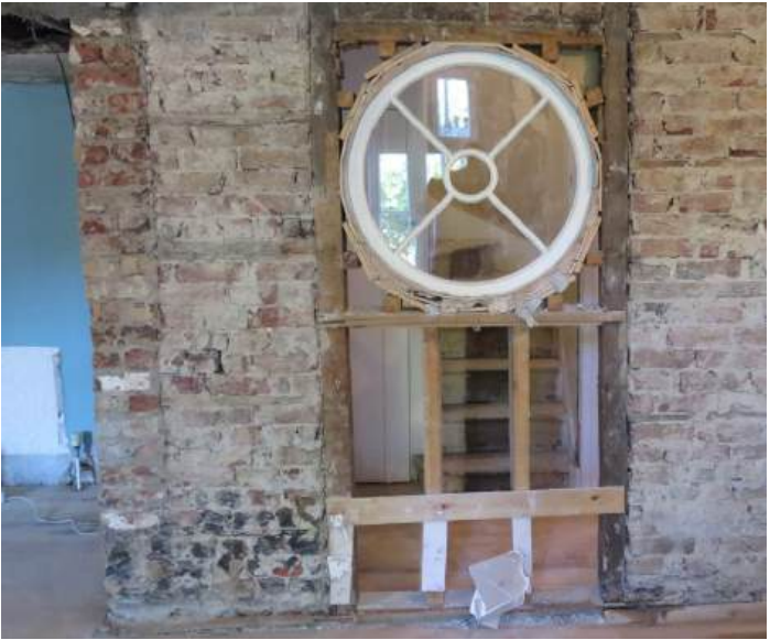
Lower ground floor - circular window added into historical door opening
