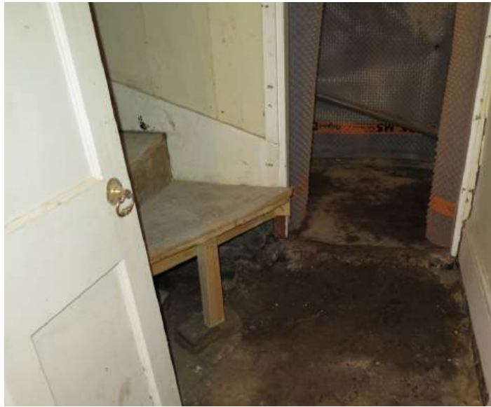
Lower ground floor main stair adaptations
