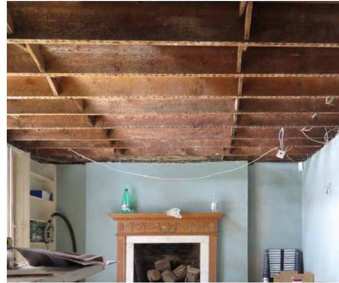
Lower ground floor central reception-original floor structure over
