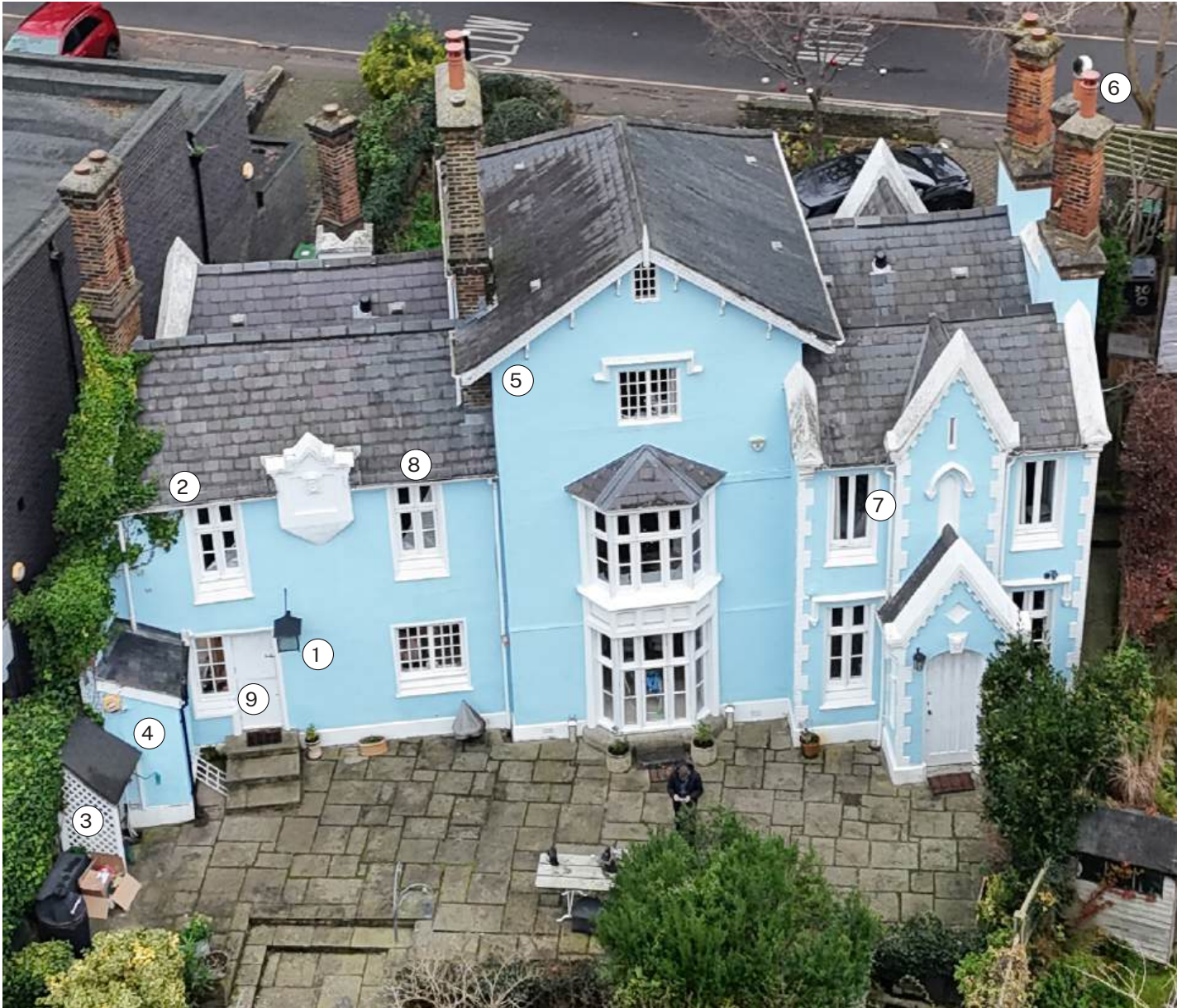
28 Wood Lane street rear elevation, image c.2014
