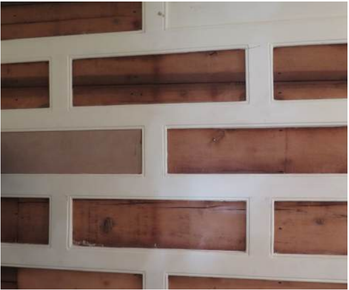
Upper ground main entrance panelling - indicative of later addition
