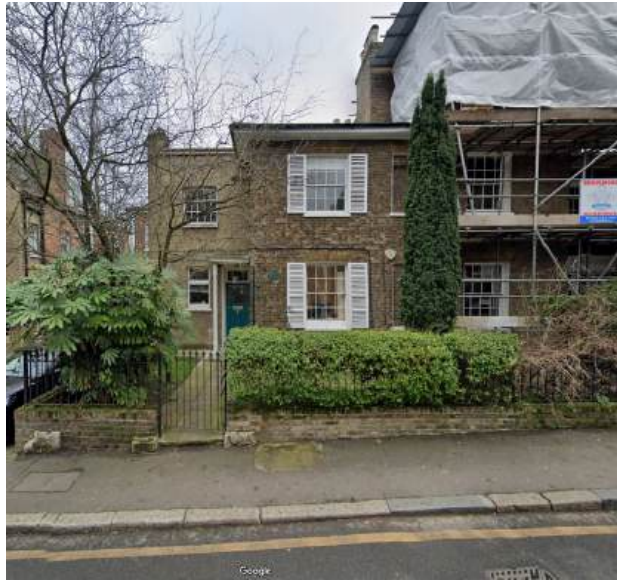
32-34 Wood Lane, Grade II listed (1816-41)
