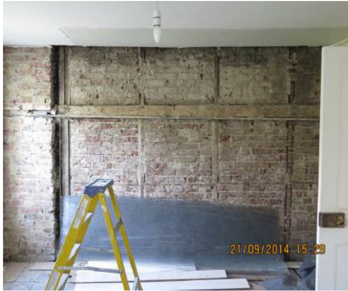
Upper ground floor east bedroom-indicating tripartite construction
