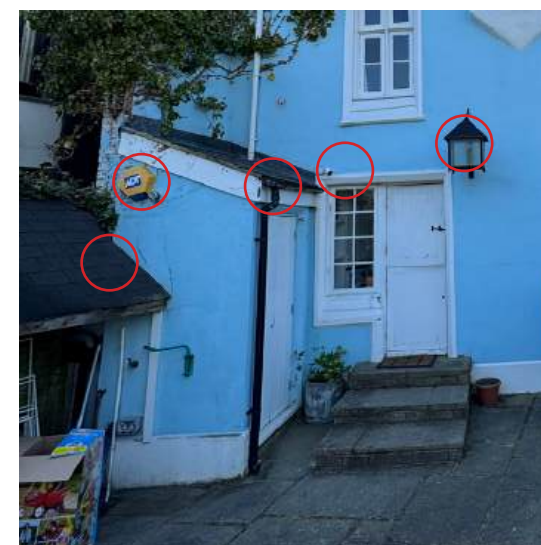
Series of images identifying external alterations to building fabric, including pipework, guttering, fascia boards and additional services
