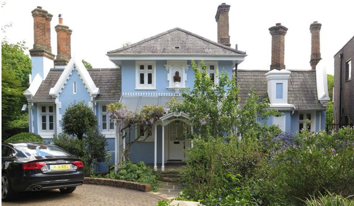
Fig.6 The main front from Wood Lane (Cooke Fawcett Architects)
