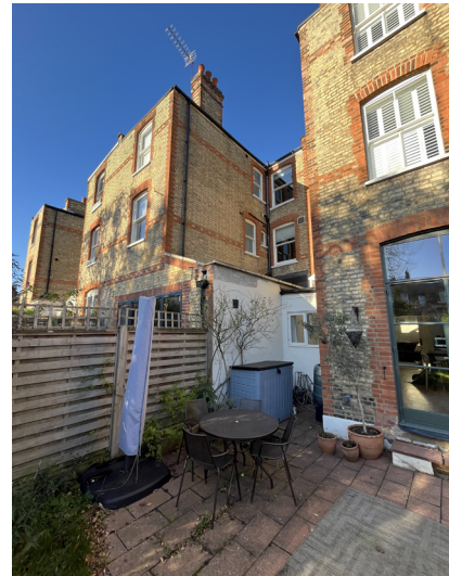
Detail of No.40 side extension / party wall
