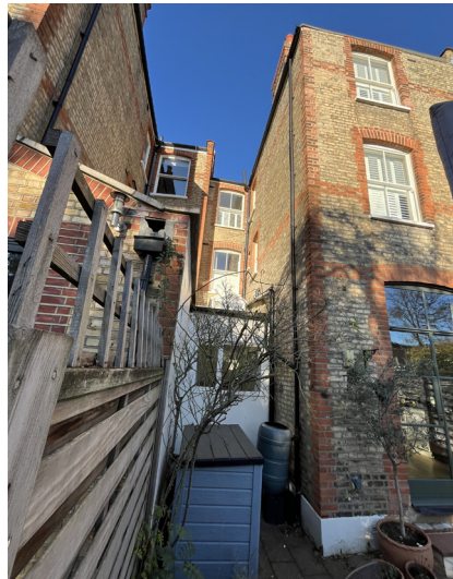
Existing side extension
