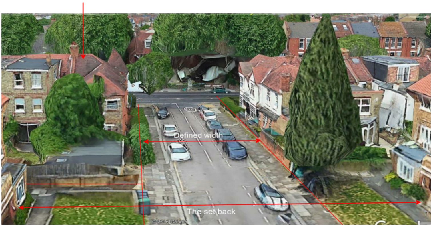
Aerial view showing the building line
