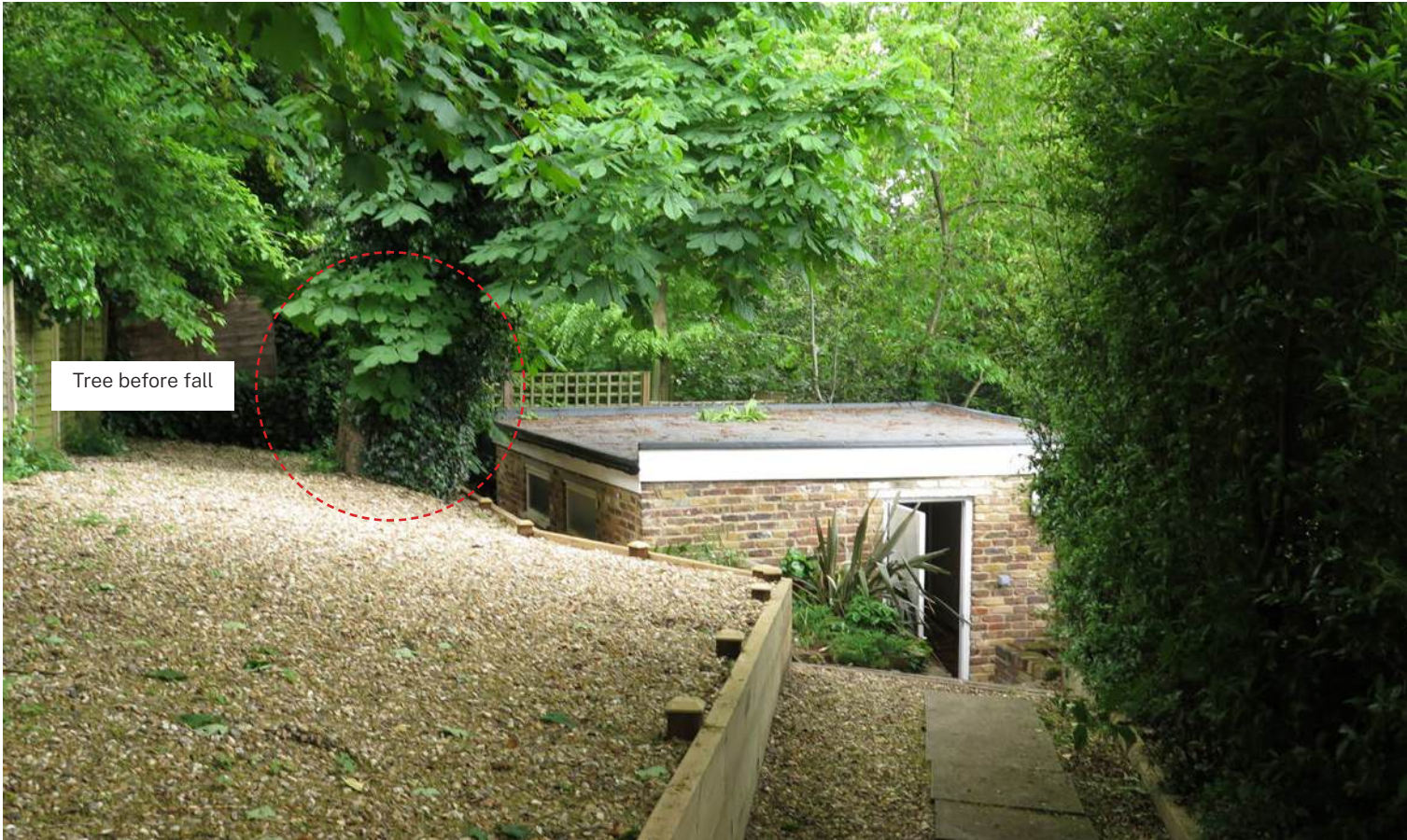
Studio before fallen tree
