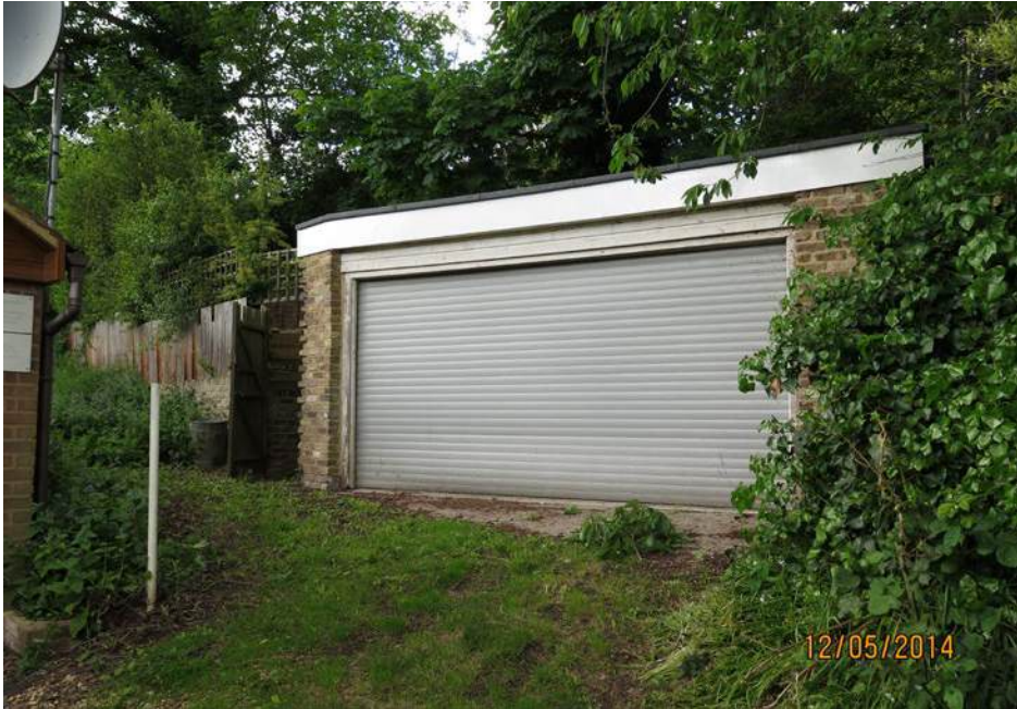
Studio before fallen tree
