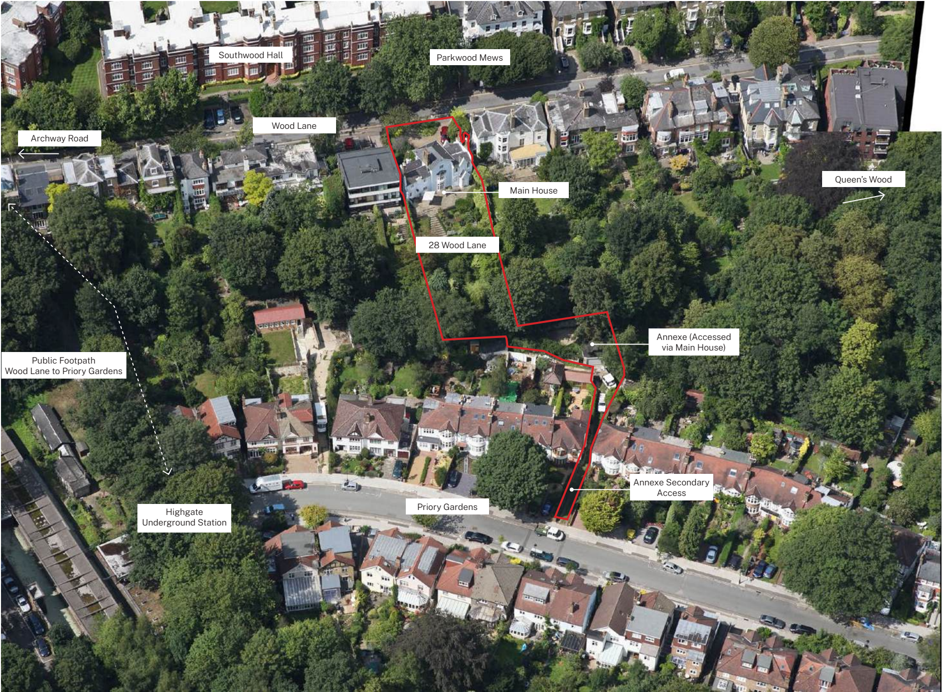
Existing Aerial View
