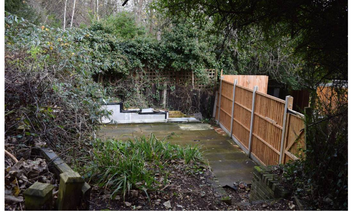
Existing studio ground slab and remaining boundary walls
