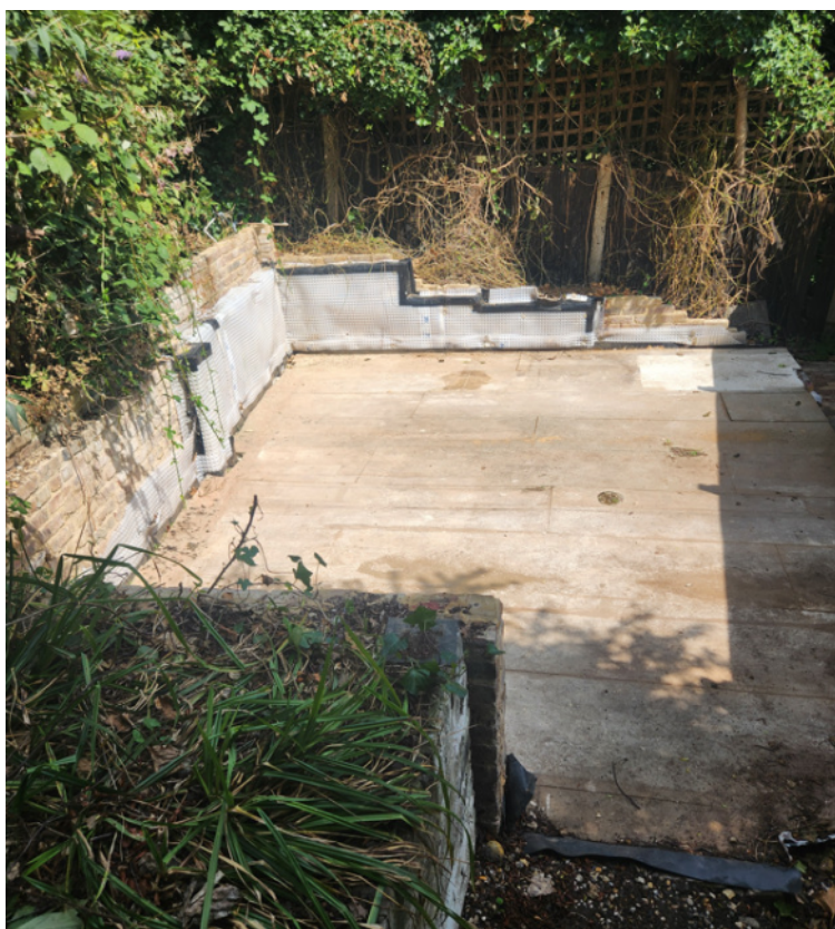
Figure 2.4 – Remnants of previous garage building to the south of the site, looking east
